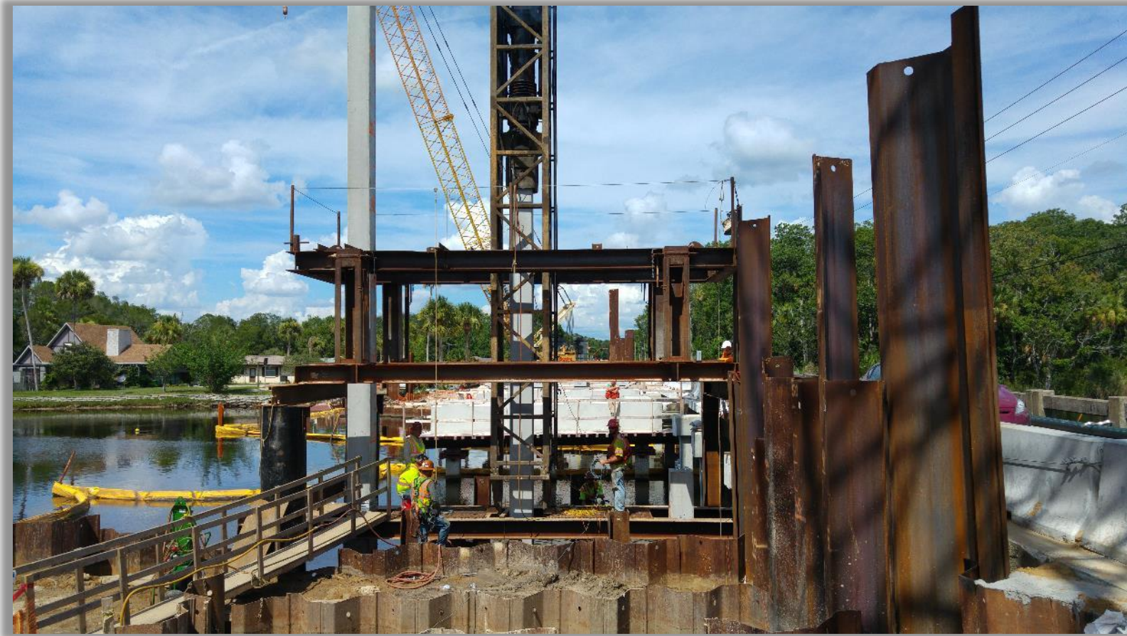
Driving of the 42 foot pile splices
