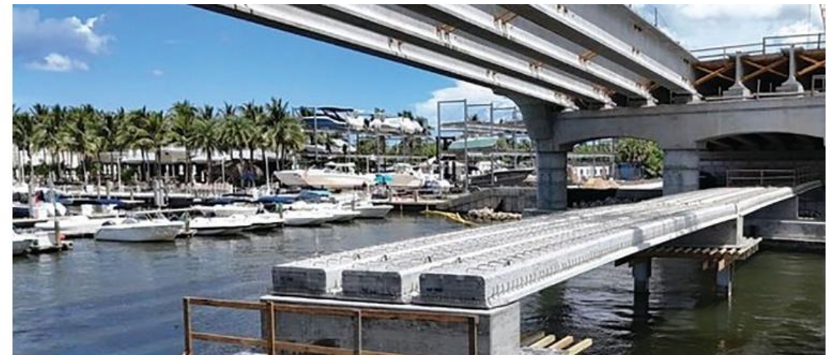
The Florida slab beams, piles, and bent caps of a low-level observation deck at the U.S. Route 1 bridge replacement in Jupiter, Fla., have carbon-fiber-reinforced-polymer prestressing strands and glass-fiber-reinforced-polymer reinforcement.
