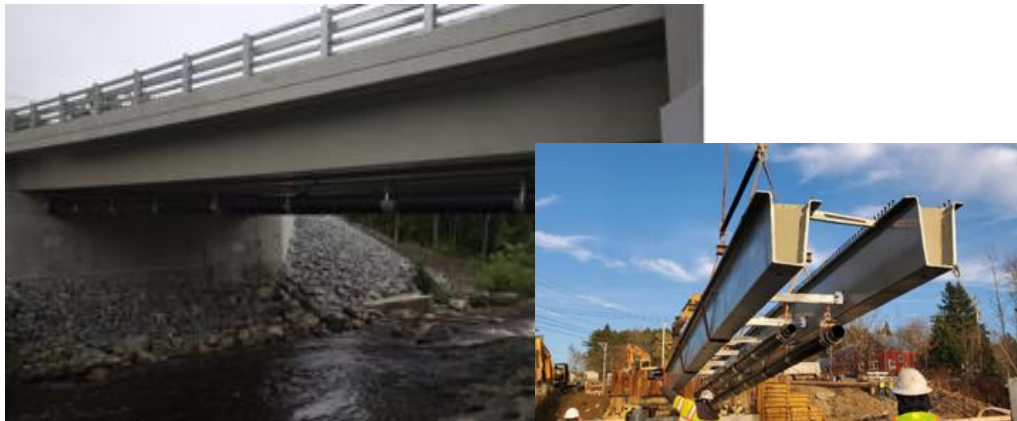
Grist Mill Bridge, Maine DOT 2021
