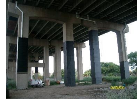
Column strengthening with CFRP wraps
