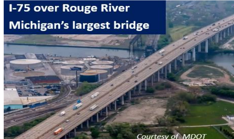
Rouge River Bridge, Michigan DOT 2019
