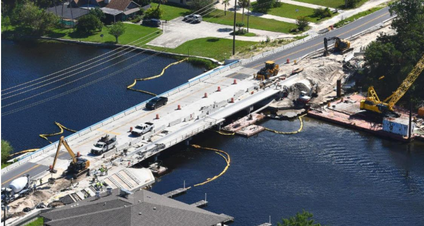
Halls River Bridge, Florida DOT 2019
