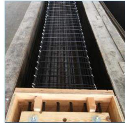
(photograph) FDOT. Wooden Headers For CFRP Strands.
