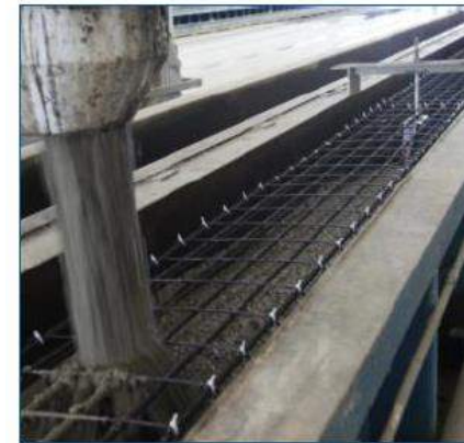
(photograph) FDOT. CFRP Pile Casting with SCC.
