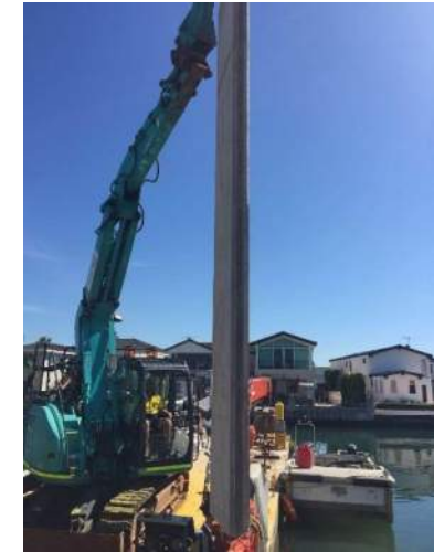
Seawall replacement, Sylvania Waters Sydney
