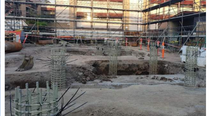
Pile cage in position
