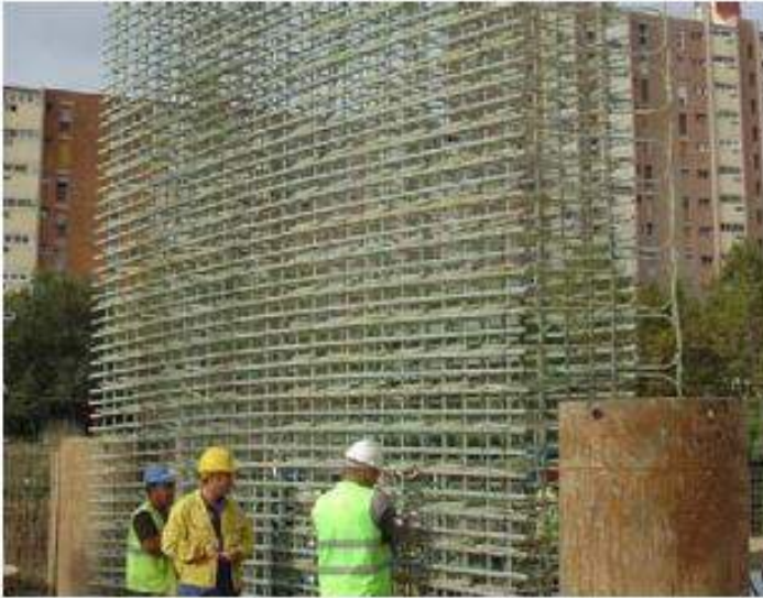
Figure 1-3: Soft eye FRP reinforcement
