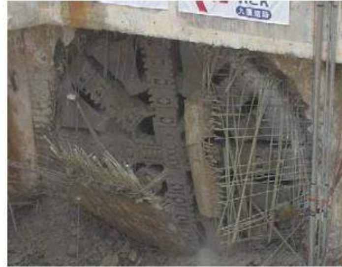
Figure 1-3: Soft eye FRP reinforcement
