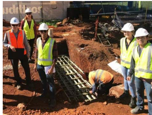
Annex extension, Toowoomba City Hall refurbishment project
