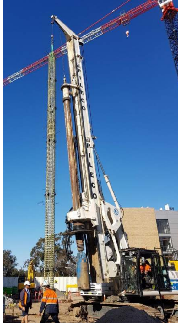
Lifting and installation of pile cage
