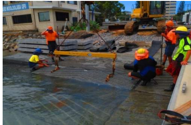
Installation of planks at Parkyn Parade boat ramp in Mooloolaba, Sunshine Coast.
