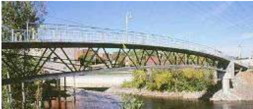
Sherbrooke pedestrian bridge
