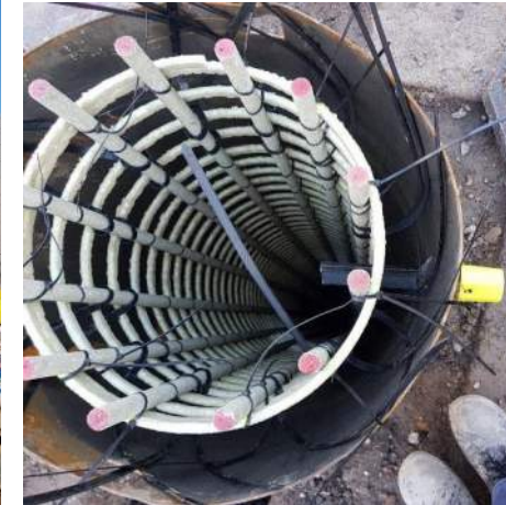
Pile cage in bored pier hole
