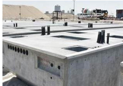
Precast concrete pontoons
