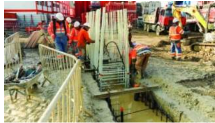
Grand Paris construction site
