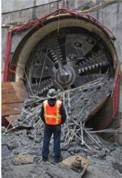
Soft-eye opening for the Bangkok Metro ( http://aslanfrp.com )
