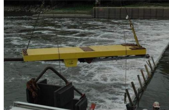
FRP composite wicket gates for IWW.
