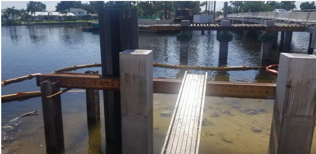
Current Construction Progress
