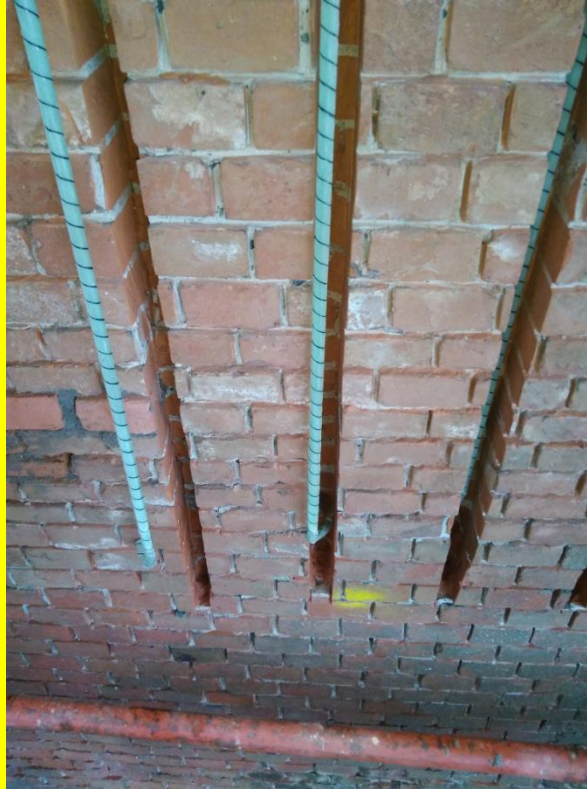
FIGURE 2: Sleeves ready for the reinforcement
