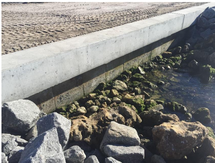
FIGURE 5. (a) Completed GFRP-RC cap on existing sheet piles
