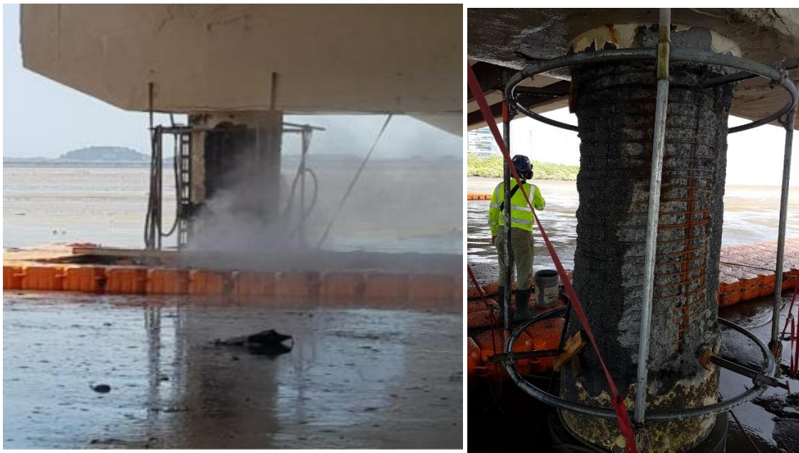
FIGURE 5: Left: hydrodemolition operation, Right: hydrodemolition frame for robotic guided nozzle
