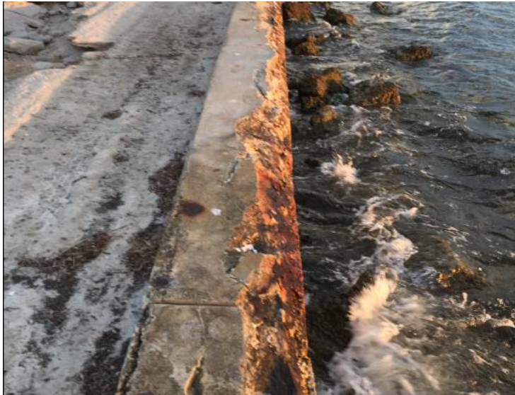
FIGURE 1. (a) Existing 1950s concrete cap to be replaced.
