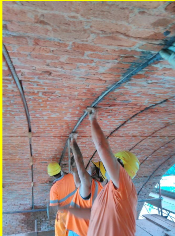
FIGURE 3: GFRP rods are inserted in the sleeves
