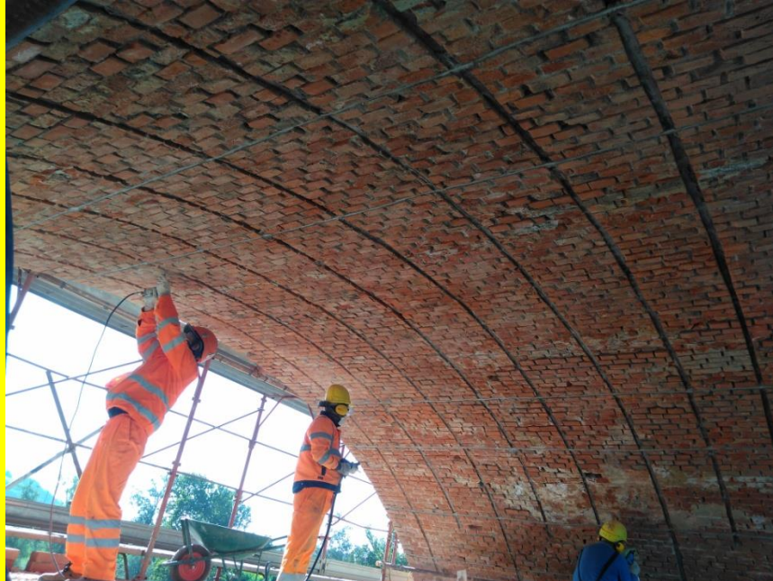
FIGURE 4: CFRP chords are applied in the transversal direction
