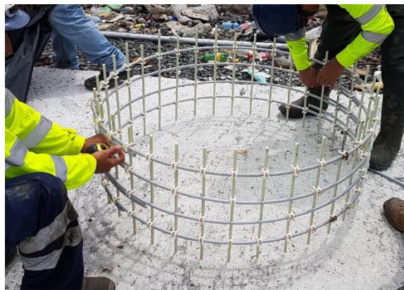
FIGURE 2: Pre-bent GFRP reinforcement for column bases
