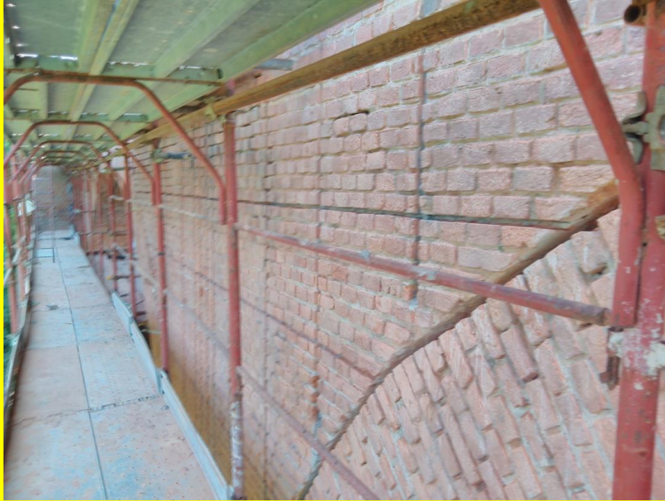
FIGURE 6: CFRP chords are travelling all around the piers
