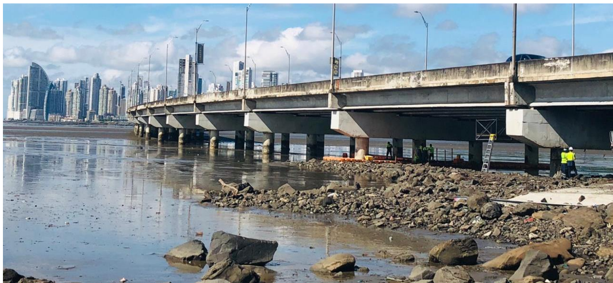
FIGURE 1: South corridor as works begin
