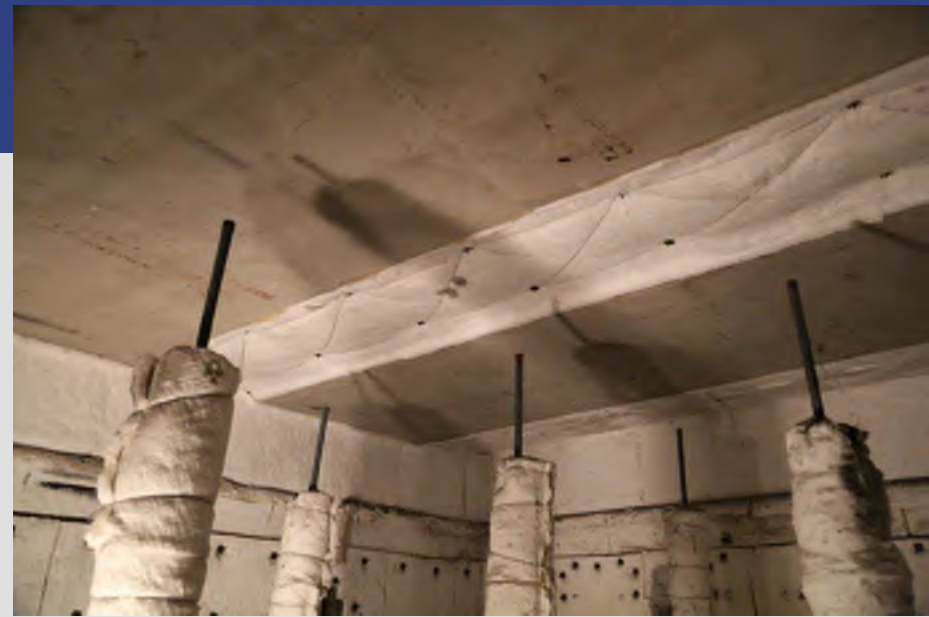
Slabs on the furnace
