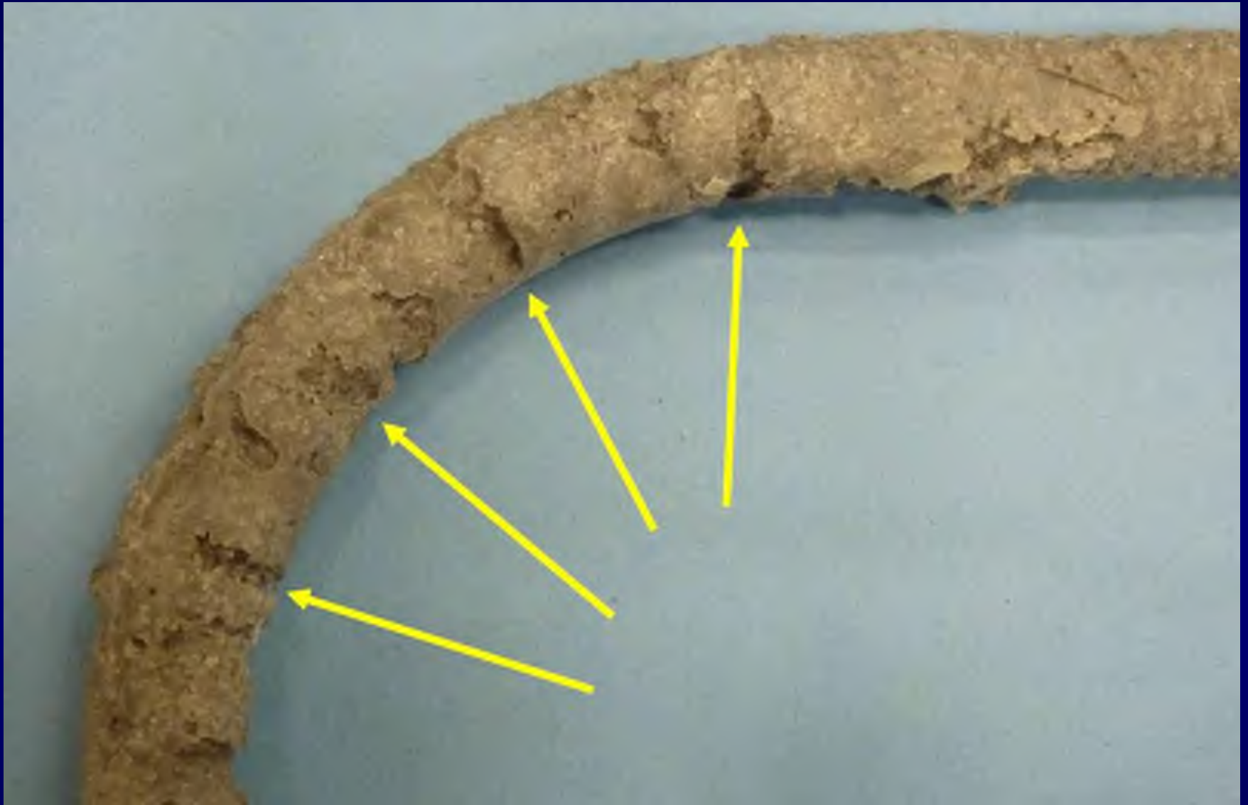
Unacceptable bar with rough, non-uniform finish and voids
