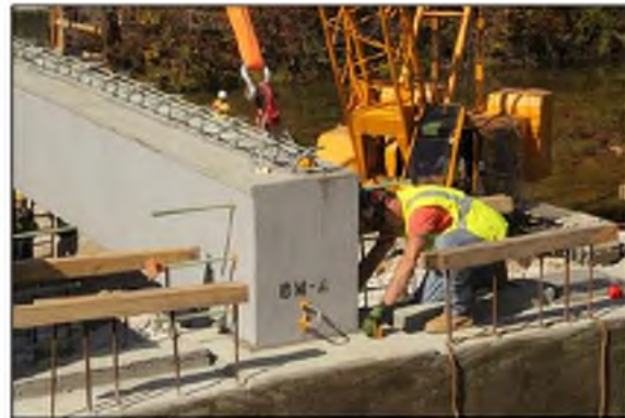
Hybrid Composite Bridge: Year 2011 Bridge built in Ava, Missouri. Use of GFRP Shell with RC Arch and Galvanized Tension Tie.
