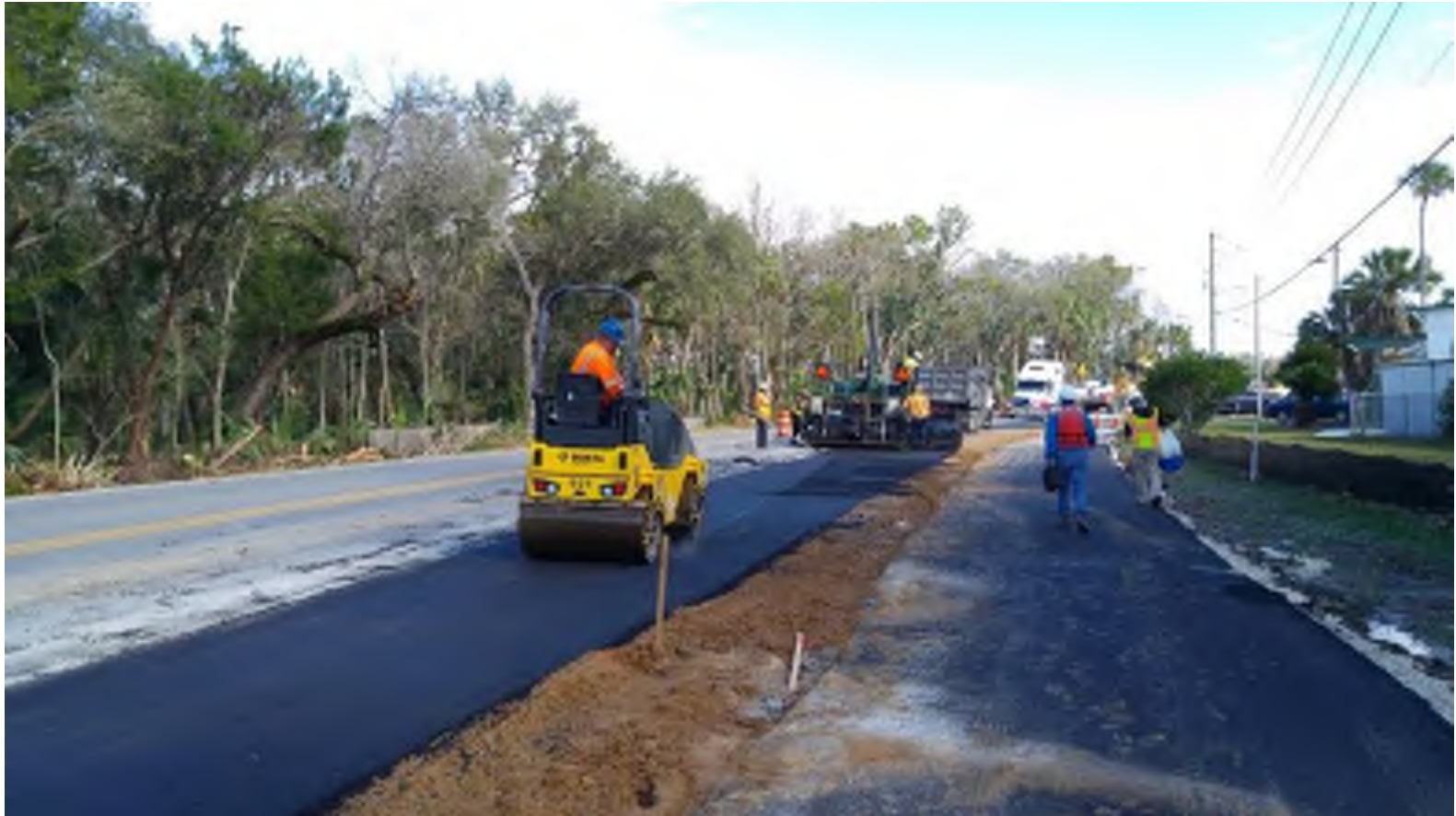
Work on approach road with temporary paving
