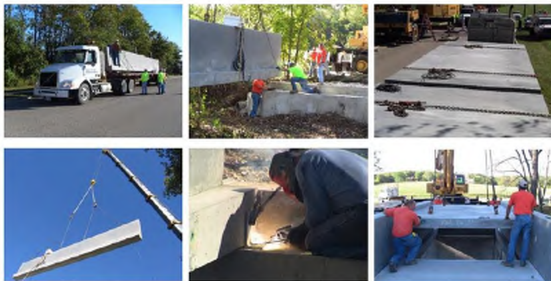
Site Installation: Two Bridges Each Erected in Less than 4 Hours
