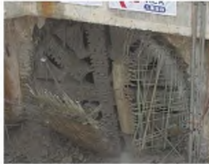
Figure 1-3: Soft eye FRP reinforcement
