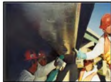
c) Conc. Repair/Putty Application
