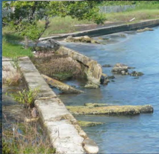
Cracking of existing seawall bulkhead cap
