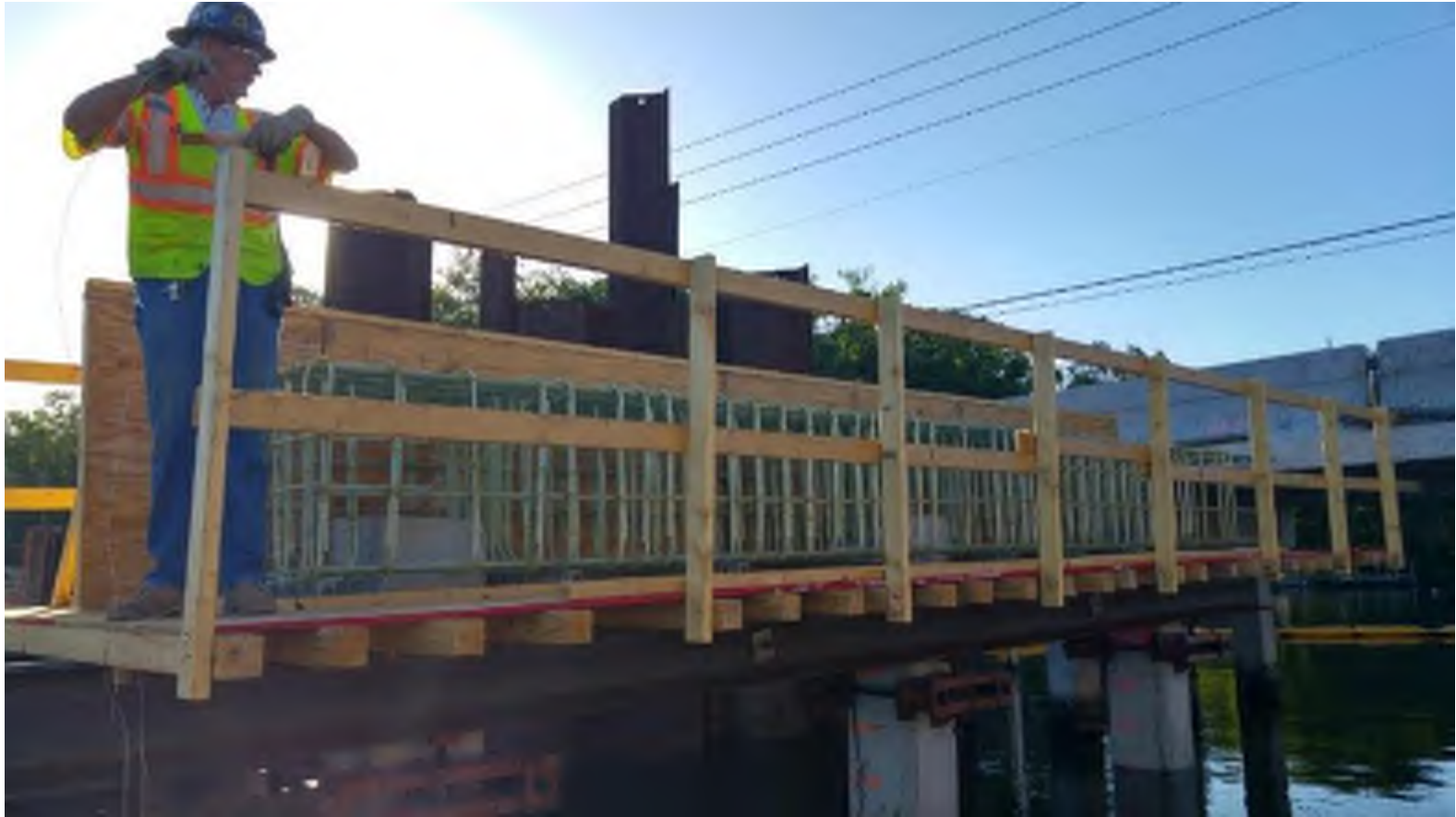
Placing of GFRP reinforcement cage at bent caps #4 and #5
