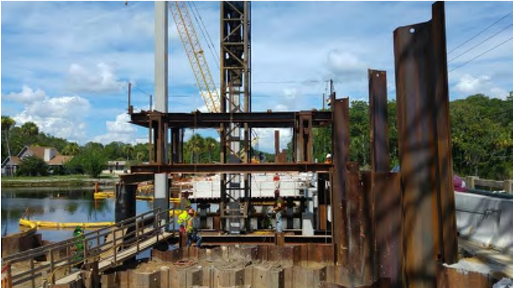
First set of the 42-ft pile splices driven in bent 2
