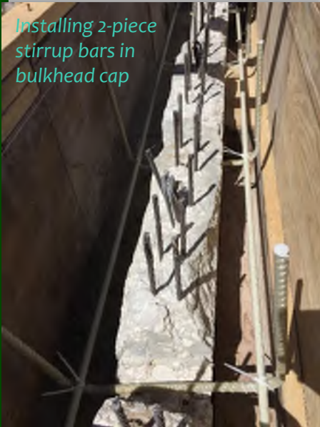
Installing 2-piece stirrup bars in bulkhead cap
