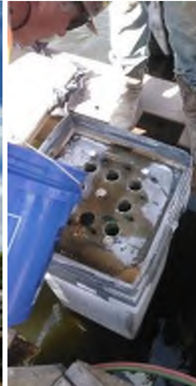
Epoxying pile splices male-female sides
