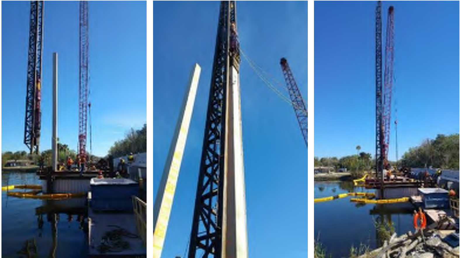
Driving of 18 in. square CFRP prestressed concrete (PC) piles at pier #3
