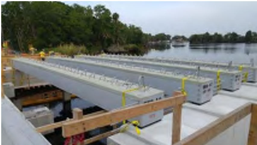
Hybrid Composite Beams set in span 4
