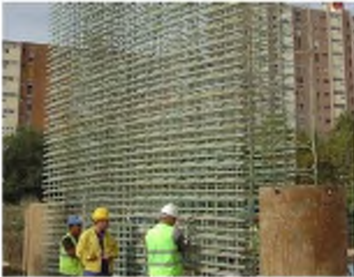
Figure 1-3: Soft eye FRP reinforcement
