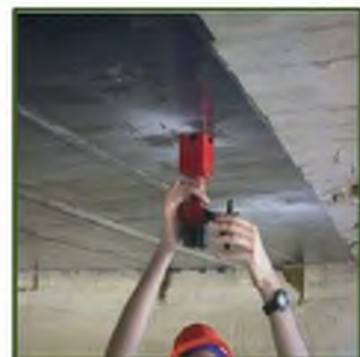
Post-Installation Bond Validation
