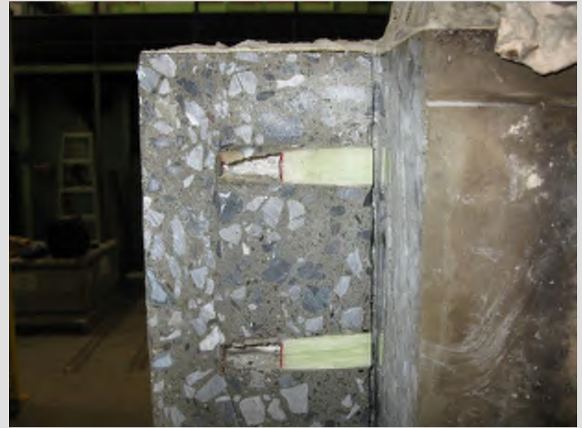
Pullout of FRP bars in the unexposed zone
