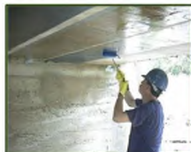
Application of Saturant and CFRP Fabric
