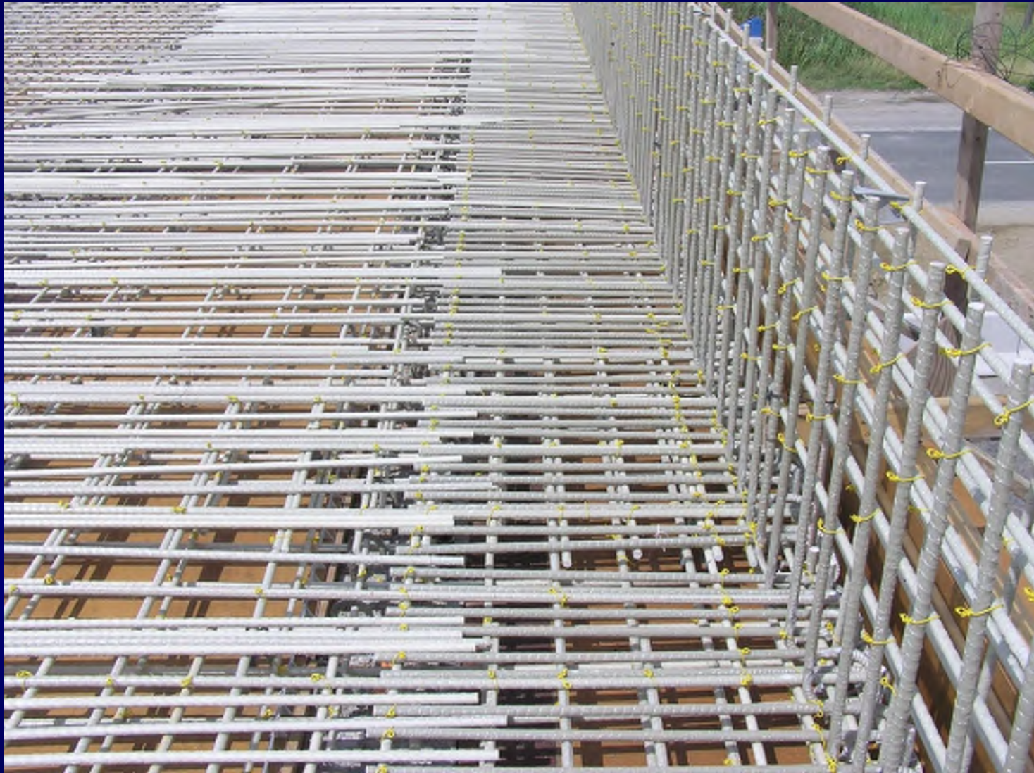
GFRP Reinforcement Top and Bottom Mat 2008
