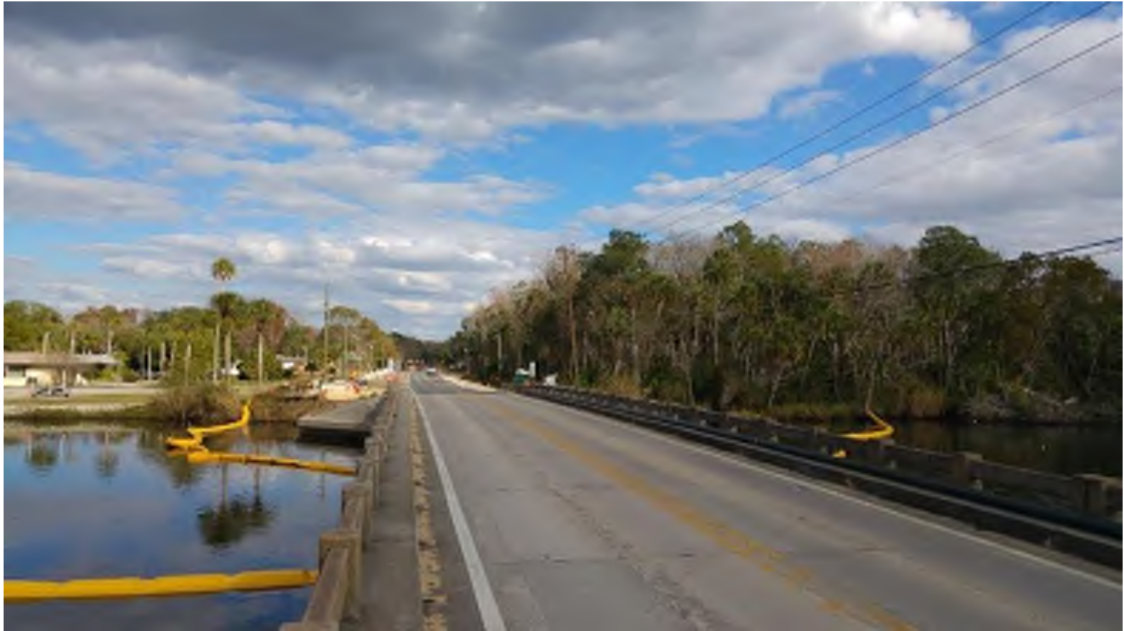
Existing bridge view
