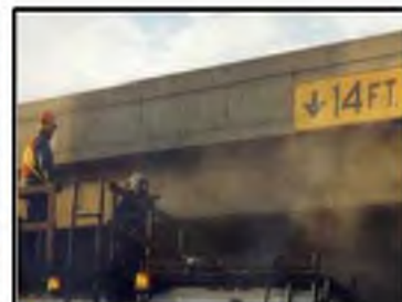
b) Surface Sandblasting
