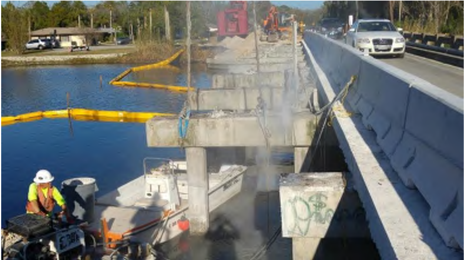
Demolition of existing bent caps and piles
