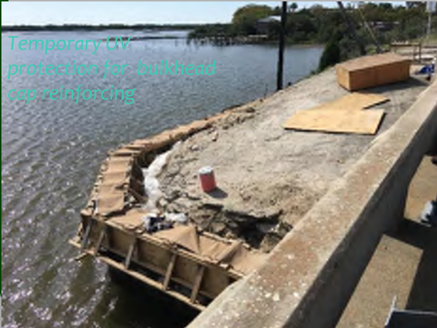
Forming bulkhead cap
