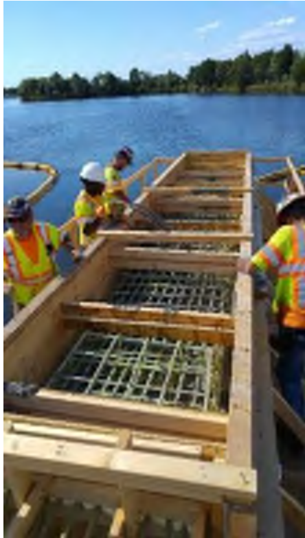
Concrete placement at bent caps #4 and #5
