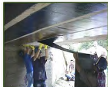
Application of Saturant and CFRP Fabric
