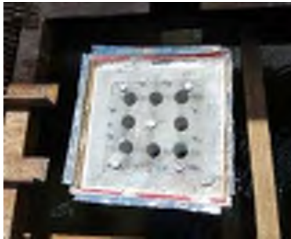
Epoxying pile splices male-female sides
