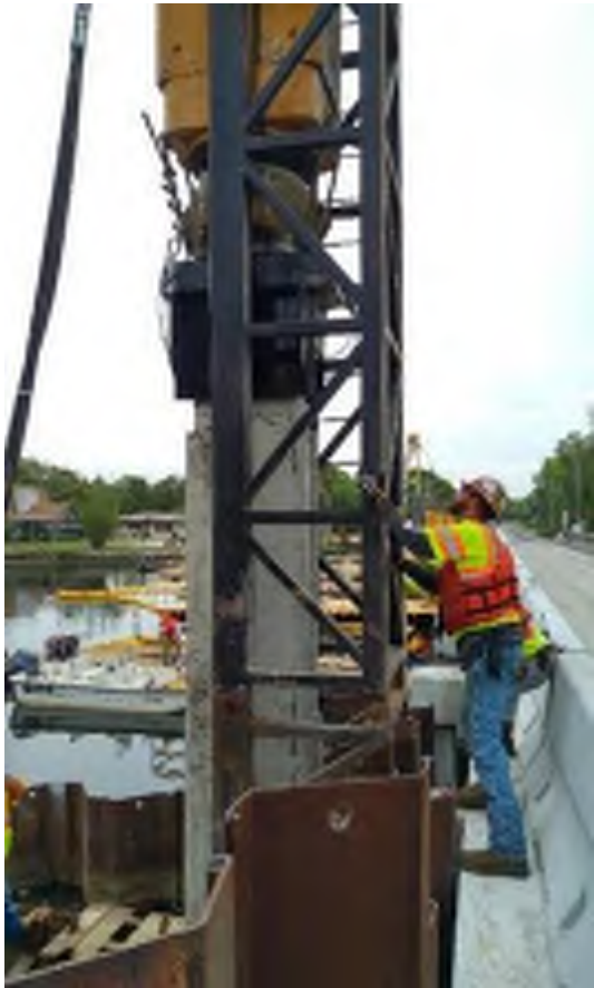
Trial installation of the CFRP-PC sheet-pile by impact hammer
