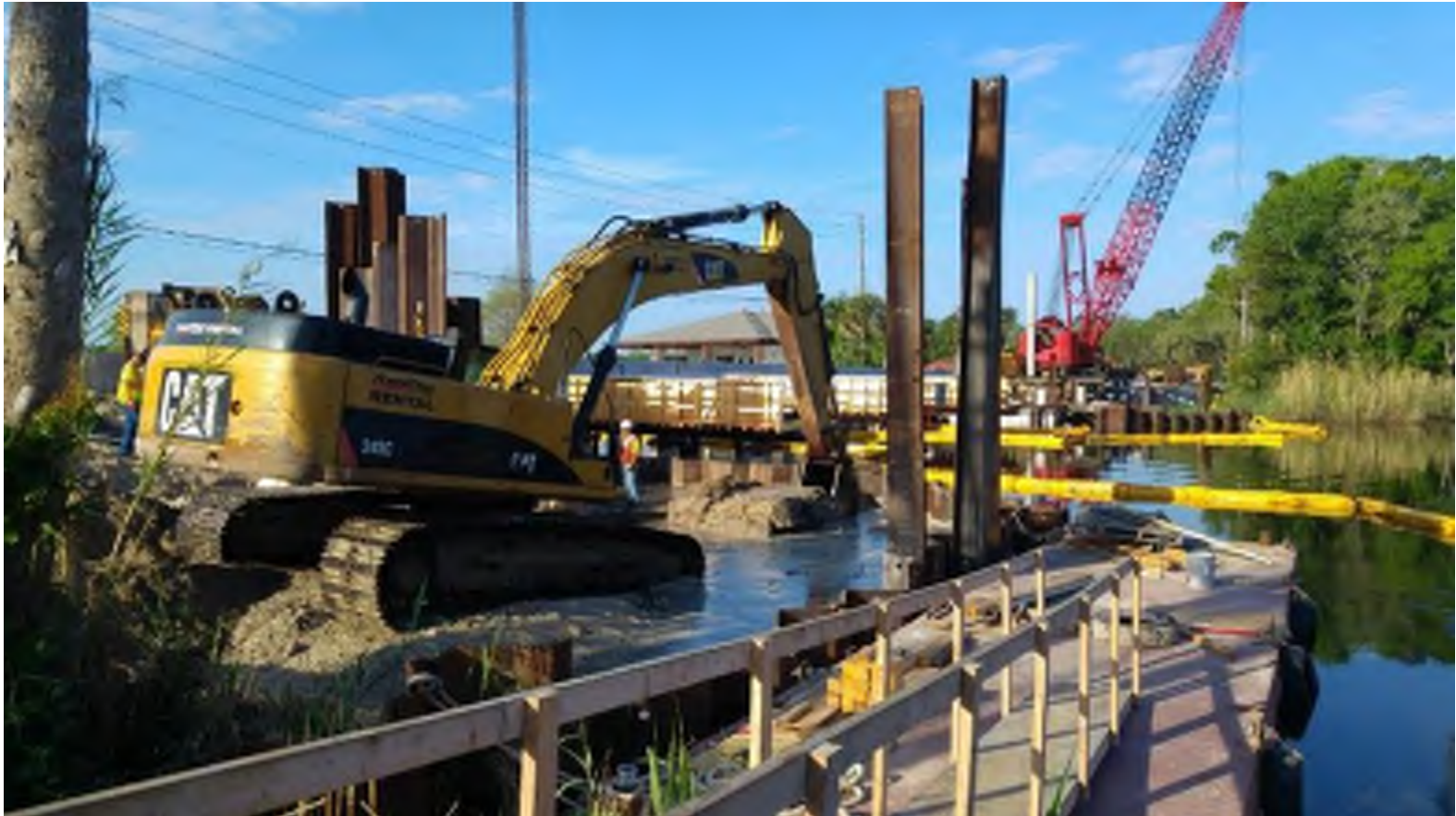
Excavation at East side for permanent CFRP-PC sheet-pile wall
