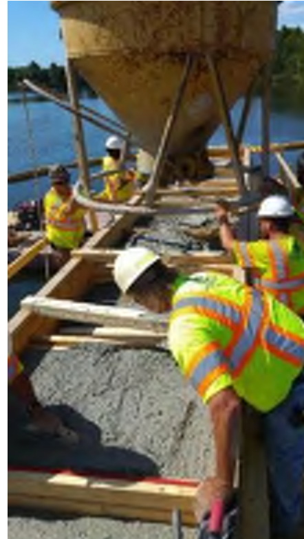
Concrete placement at bent caps #4 and #5
