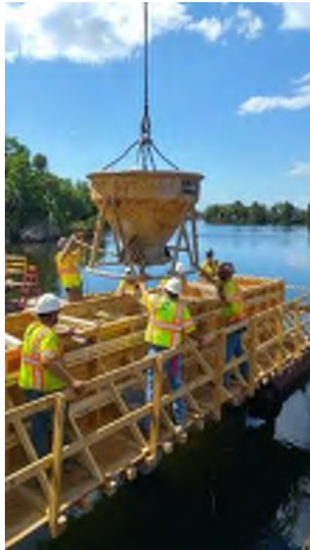
Concrete placement at bent caps #4 and #5
