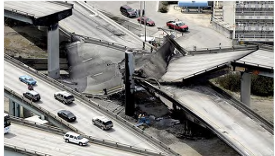
An aerial view of the collapsed freeway overpass near downtown Oakland
