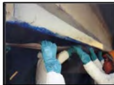
e) Manual Lay-up of CFRP Sheet
