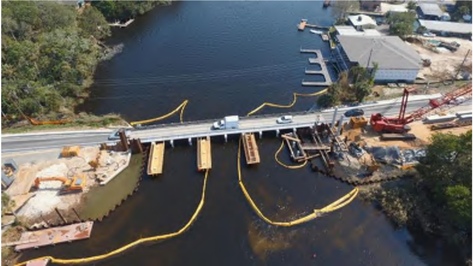
View of formwork and temporary sheet-pile installation on the East side
