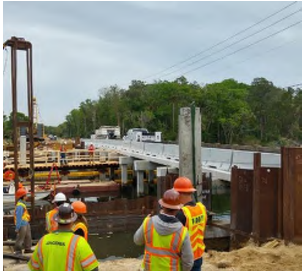
Trial installation of the CFRP-PC sheet-pile by impact hammer
