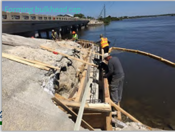
Installing 2-piece stirrup bars in bulkhead cap
