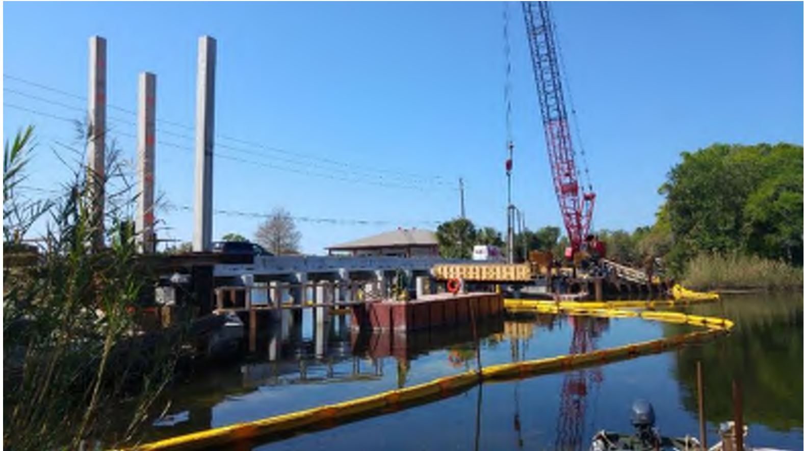
Piles driven at piers #4 and #6
