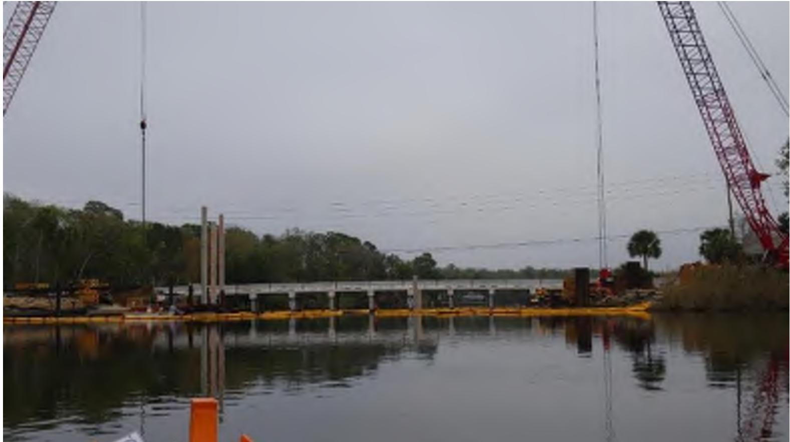
Piles driven at piers #3 and #5; temporary sheet-pile installation at West side
