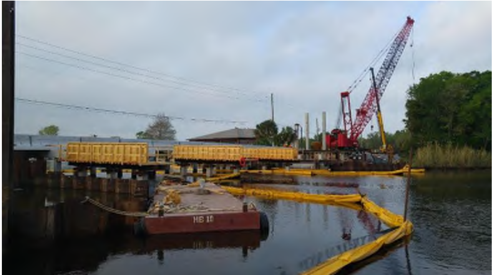
Formwork installation for bent caps at piers #3, #4 and #5
