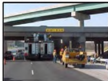
a) Overall View
