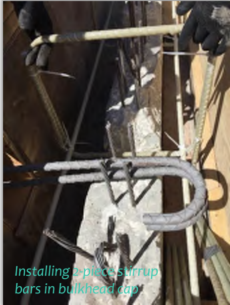
Forming bulkhead cap
