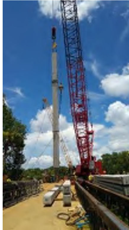
Epoxying pile splices male-female sides
