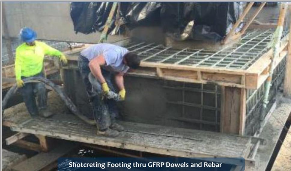
Shotcreting Footing thru GFRP Dowels and Rebar
