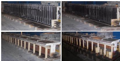
Reinforcing Cage and Concrete Casting
