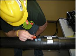
Check for gaps and visible wires Figure 21
