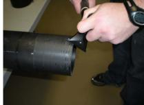
Deburring or Beveling pipe ends Figure 10
