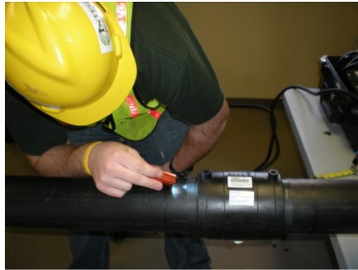
**Check for gaps and visible wires
