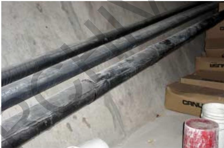
*Figure 4.2 – Heat Activated Adhesive Duct Wrapping for External Post-tensioning Tendons*
