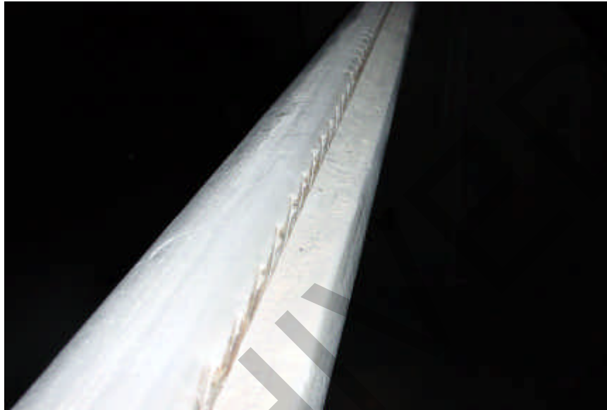
Figure 2.1 – Bleed water trail in Tendon 37-4 found by sounding inspection.
