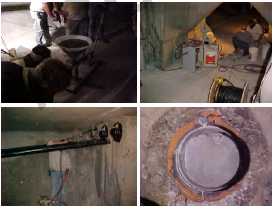
Figure 2.13 – Field trial of the vacuum injection method.
