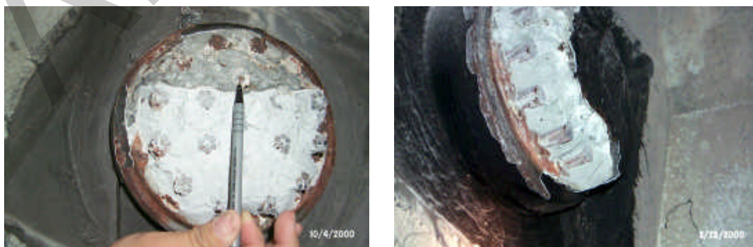
Figure 3.4 – Secondary Grout in Anchor Caps
