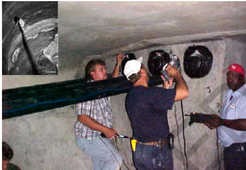
Figure 2.3 – Borescope Inspection of a Post-Tensioning Tendon Anchor.
