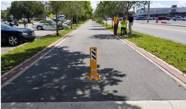
Figure 4: Site Evaluation with City of Gainesville. The team observed numerous shared-use paths leading in and out of the University of Florida.
