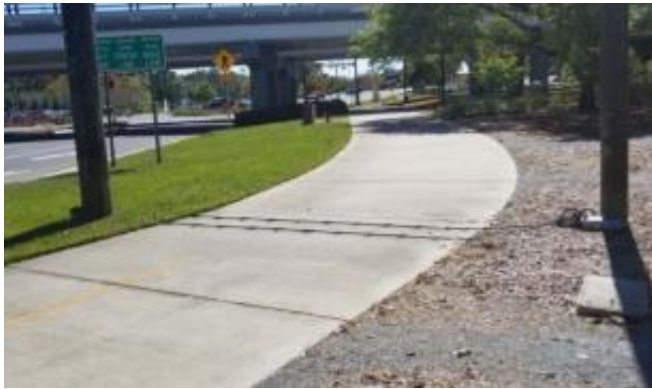
Figure 16: Technicians utilize poles, signs, and trees as potential features to attach the lock for the count device.
