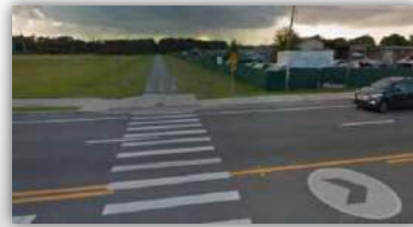
Site selected for Potential Continuous Bicycle /Pedestrian Counting Shingle Creek Trail, Kissimmee, Florida
