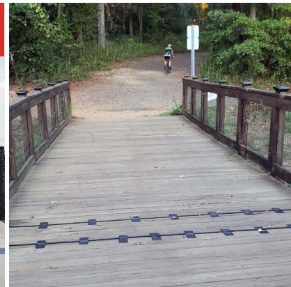
Lafayette Bridge Count | Tallahassee, FL
