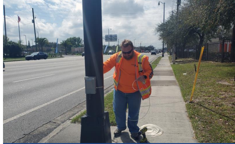
Short-term count installation in Seminole County
