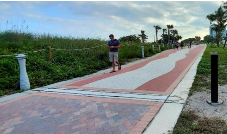
Recent continuous count station installation along Atlantic Greenway Trail in Miami Beach
