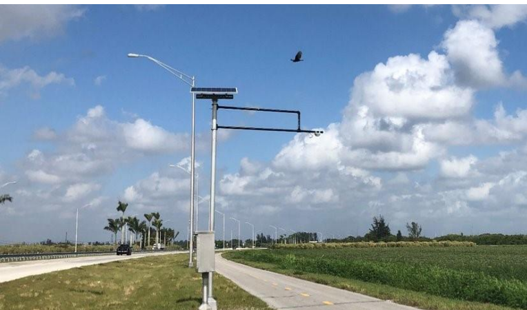
Recent continuous count station installation along Krome Path in West Kendall community / unincorporated Miami-Dade County
