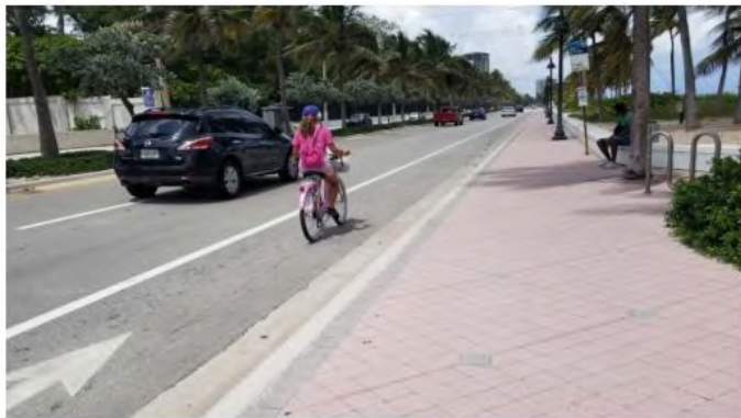
Site Visit Photos:
