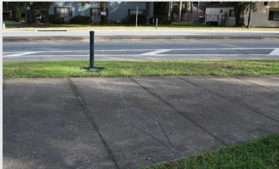
Eco-Counter side detection passive infrared with loops
