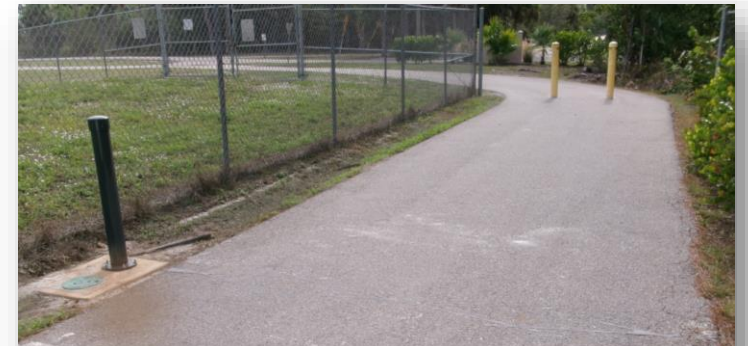
Gordon River Greenway, Naples, Collier County Side Fire Infrared with Inductive Loops 2023 Avg. Daily Users: 740
