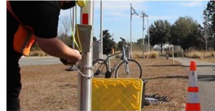
Figure 65: Non-Motorized Infrared Deployment Lock and Chain
