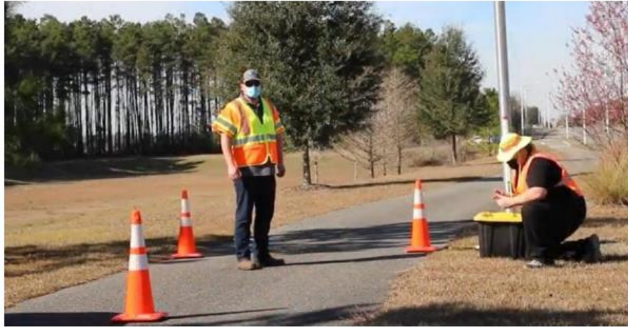
Figure 63: Non-Motorized Deployment Work zone
