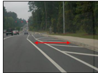
2 – Paved with Warning Device
