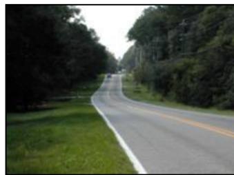
4 – Passing restrictions due to grades on over 50% of sample length
