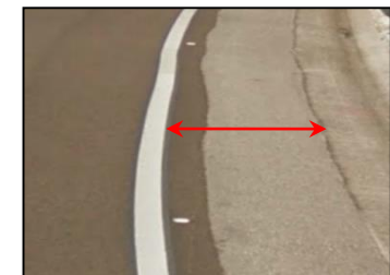
2 – Paved with Warning Device
