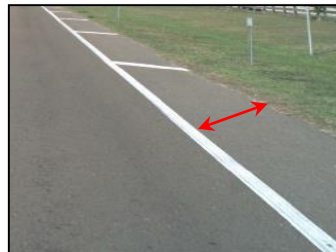
2 – Paved with Warning Device
