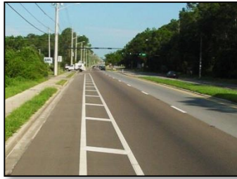
Perpendicular to roadway
