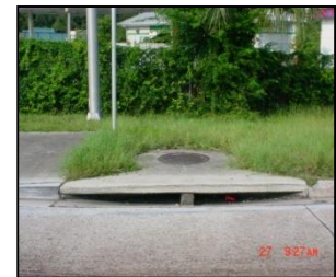
Curb inlet with manhole
