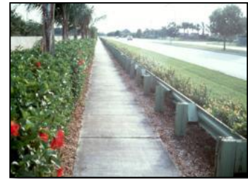
4 – Guardrail/traffic railing barrier
