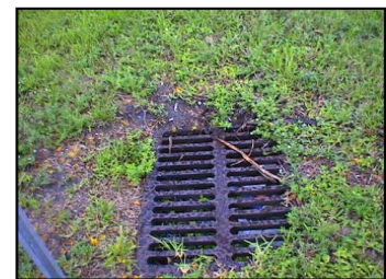
In ditch bottom
