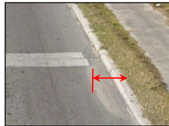
8 – Curb with Resurfaced Gutter
