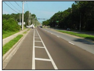
Perpendicular to Roadway
