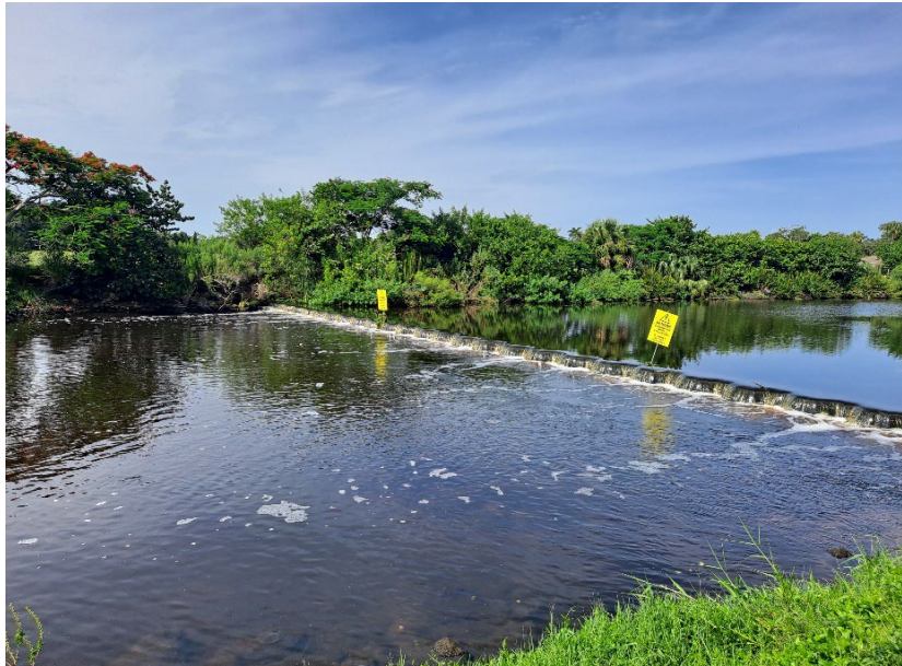
Representative 8160 - Salinity control structure east of study area
