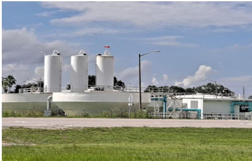
Representative 8340 - Wastewater Treatment Plant
