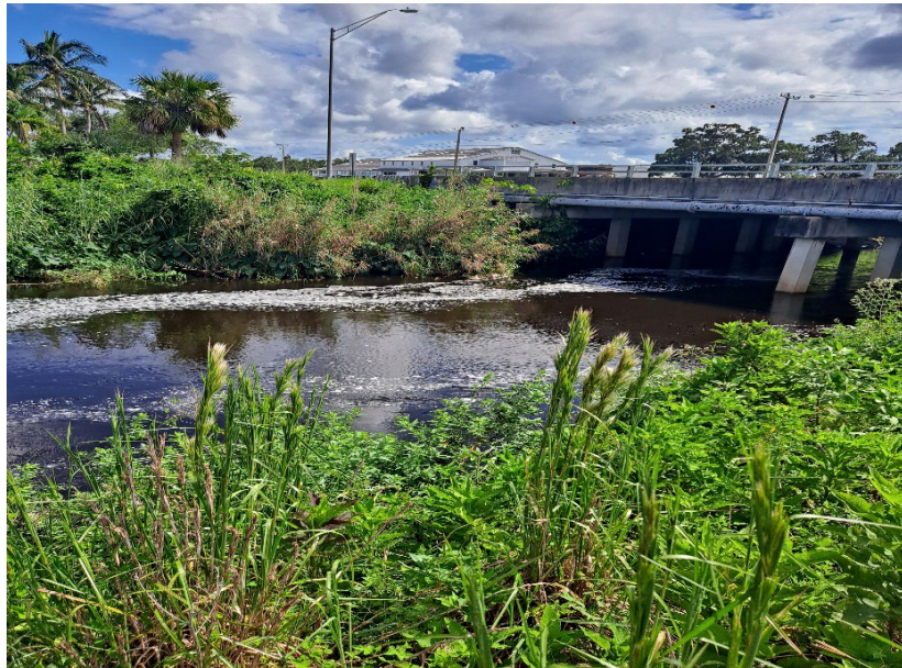
Representative 5100 - Streams and Waterways (Main Canal)
