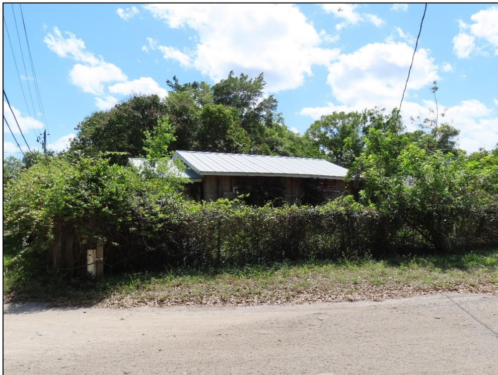
Figure 60: 3245 13 th Avenue (8IR1886), c. 1946, Considered National Register-Ineligible, facing South
