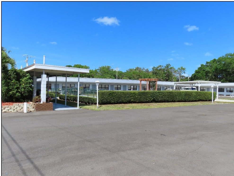
Figure 57: 3256 US 1 (8IR1883), c. 1955, Considered National Register-Ineligible, facing Northeast
