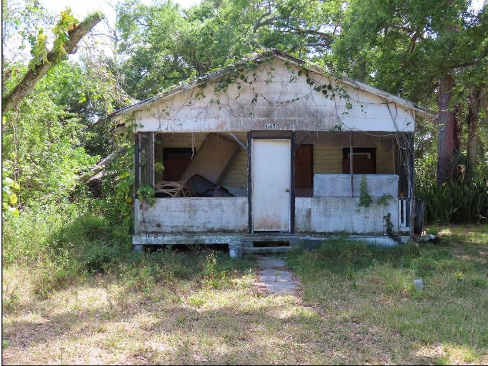
Figure 48: 1365 33 rd Street (8IR762), c. 1934, Considered National Register-Ineligible, facing South
