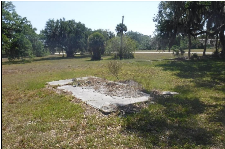
Figure 24: Concrete slab in a vacant lot north of 30 th Street and East of US 1, in Proposed Pond 1A, facing Southeast
