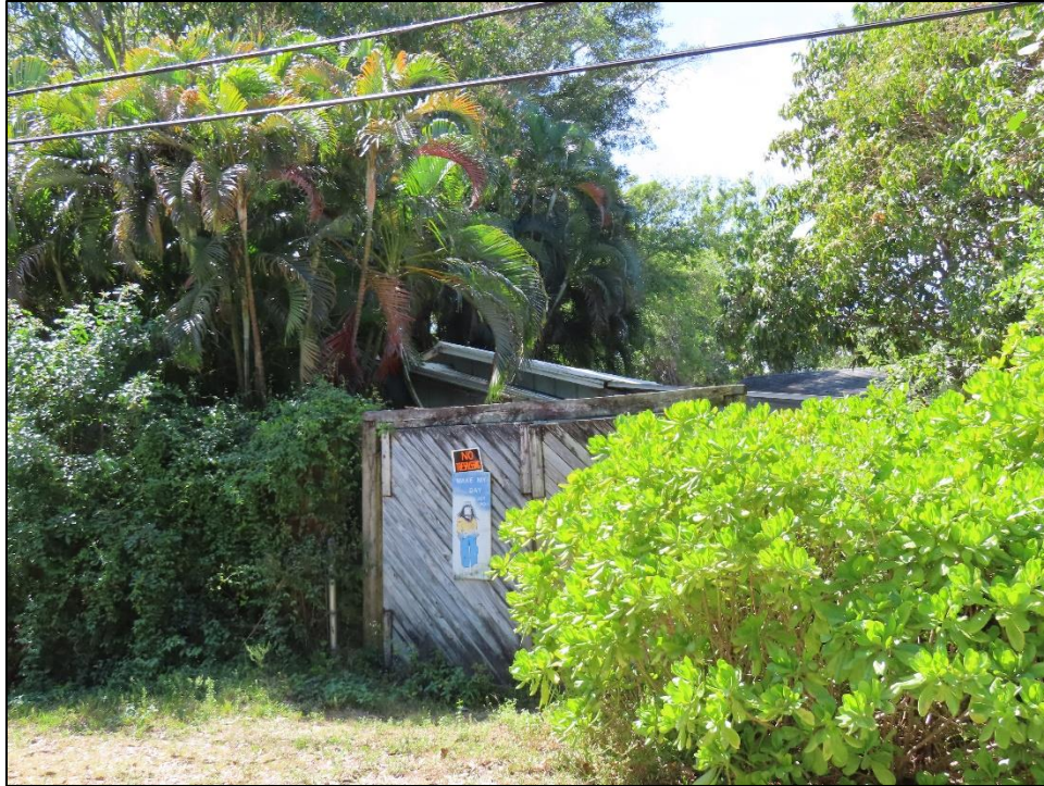
Figure 77: 3235 13 th Avenue (8IR1900), c. 1940, Considered National Register-Ineligible, facing West
