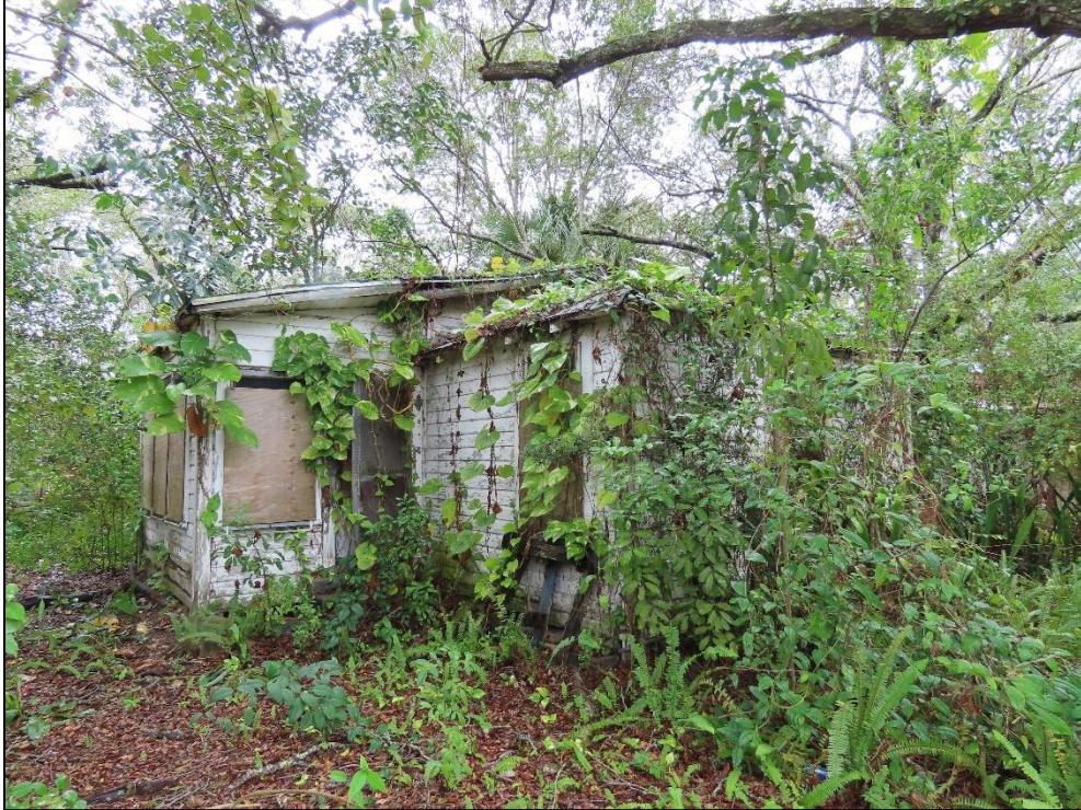
Figure 41: 1336 32 nd Street (8IR750), c. 1935, Considered National Register-Ineligible, facing Northeast
