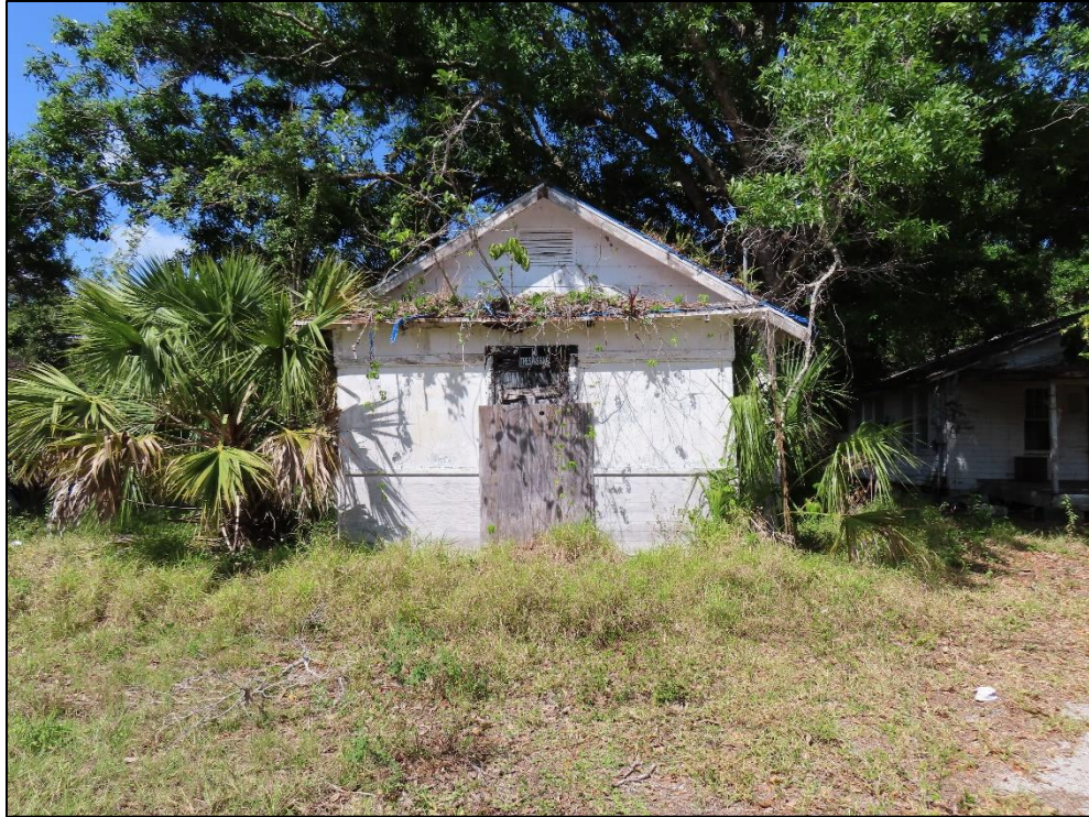
Figure 47: 1326 33 rd Street (8IR758), c. 1920, Considered National Register-Ineligible, facing North
