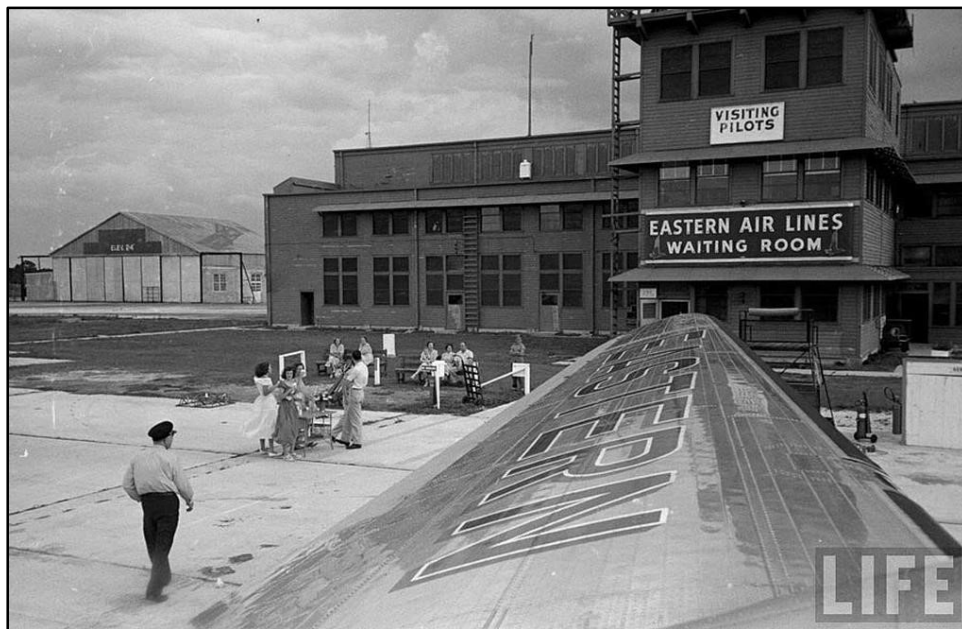
Figure 3: A 1949 Photo of the Terminal Building ( Sunshine Skies )
