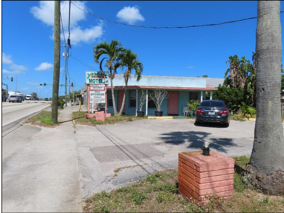
Figure 84: Vero's Motel Complex (8IR1904), c. 1951, Considered National Register-Ineligible, facing North
