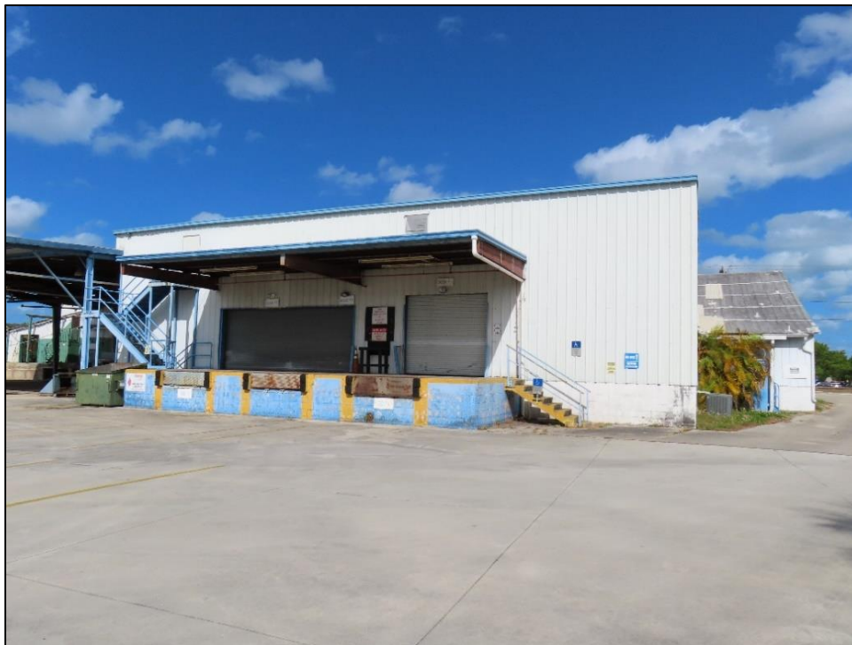
Figure 69: 2745 St. Lucie Avenue (8IR1894) Southwestern Addition, c. 1974, Considered National Register-Eligible, facing East
