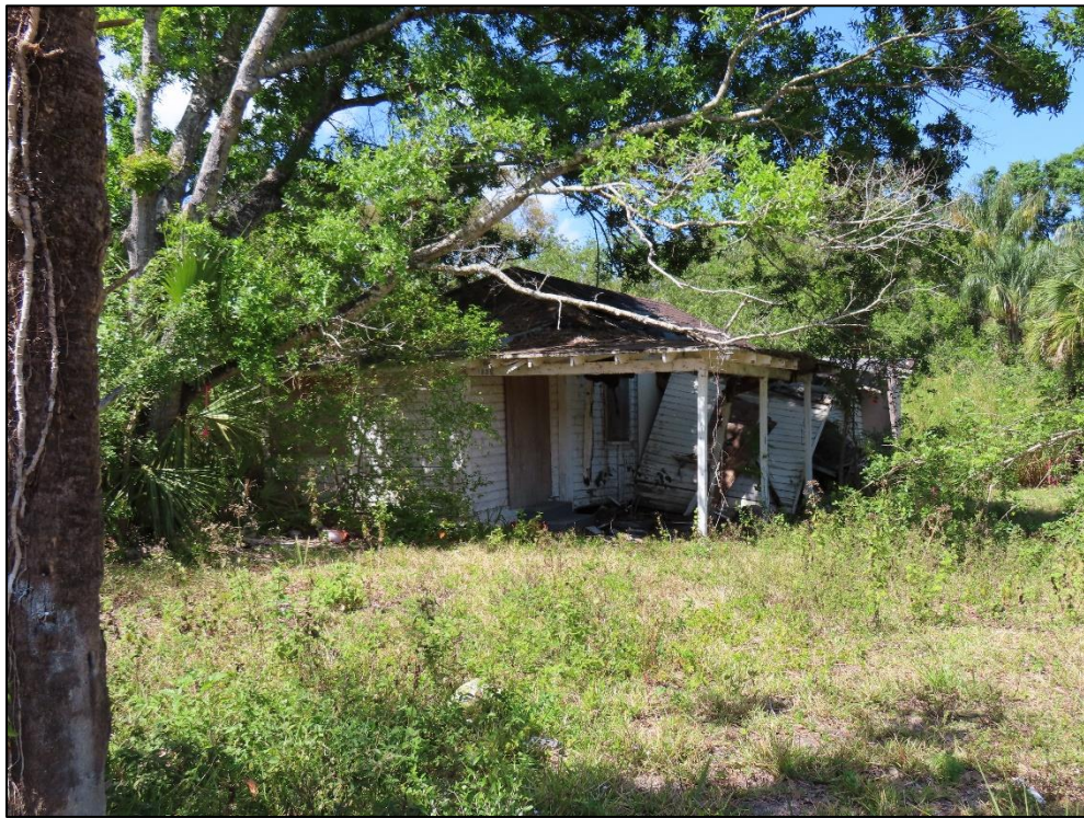
Figure 59: 1336 33 rd Street (8IR1885), c. 1928, Considered National Register-Ineligible, facing North
