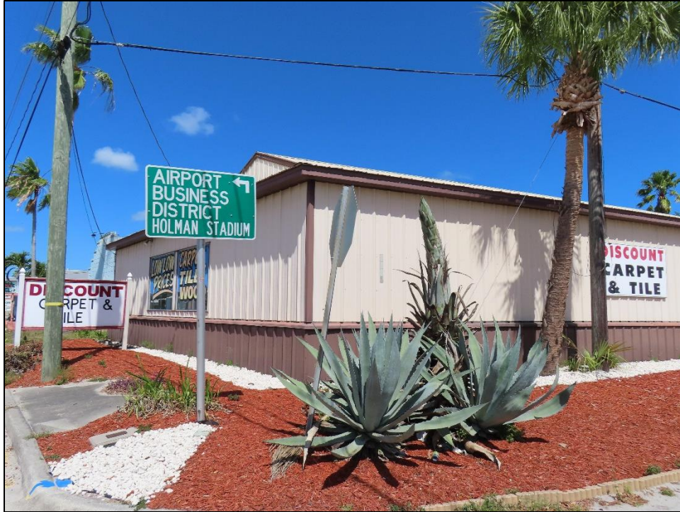
Figure 78: 3106 US Highway 1 (8IR1901), c. 1935, Considered National Register-Ineligible, facing Northeast
