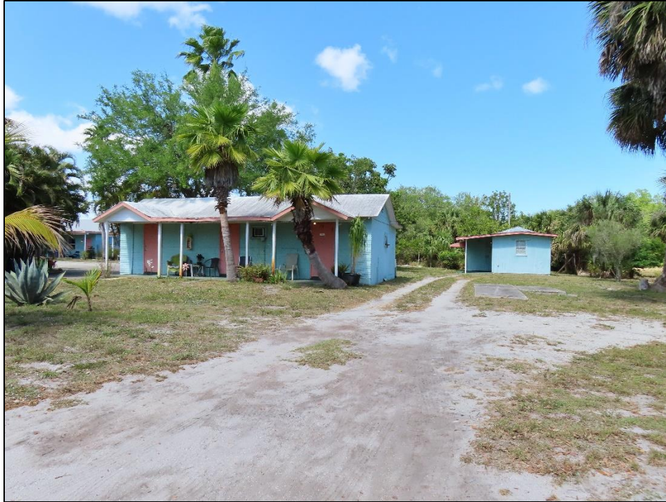
Figure 88: Vero's Motel Complex (8IR1904), c. 1951, Considered National Register-Ineligible, facing North
