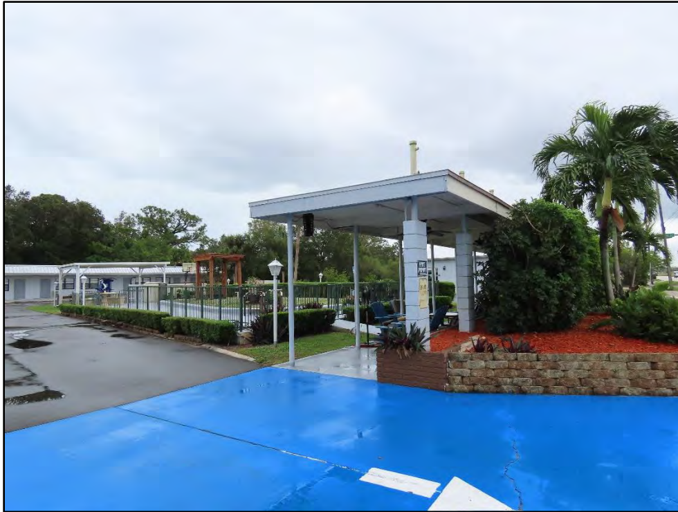
Figure 3: 3256 US 1 (8IR1883), facing Southeast
