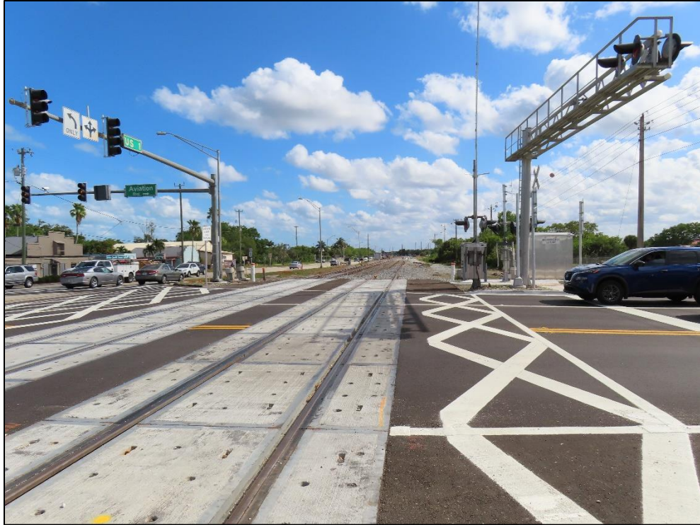
Figure 53: FEC Railway (8IR1497), c. 1892, Determined National Register-Eligible, From Intersection with Aviation Boulevard, facing Southeast
