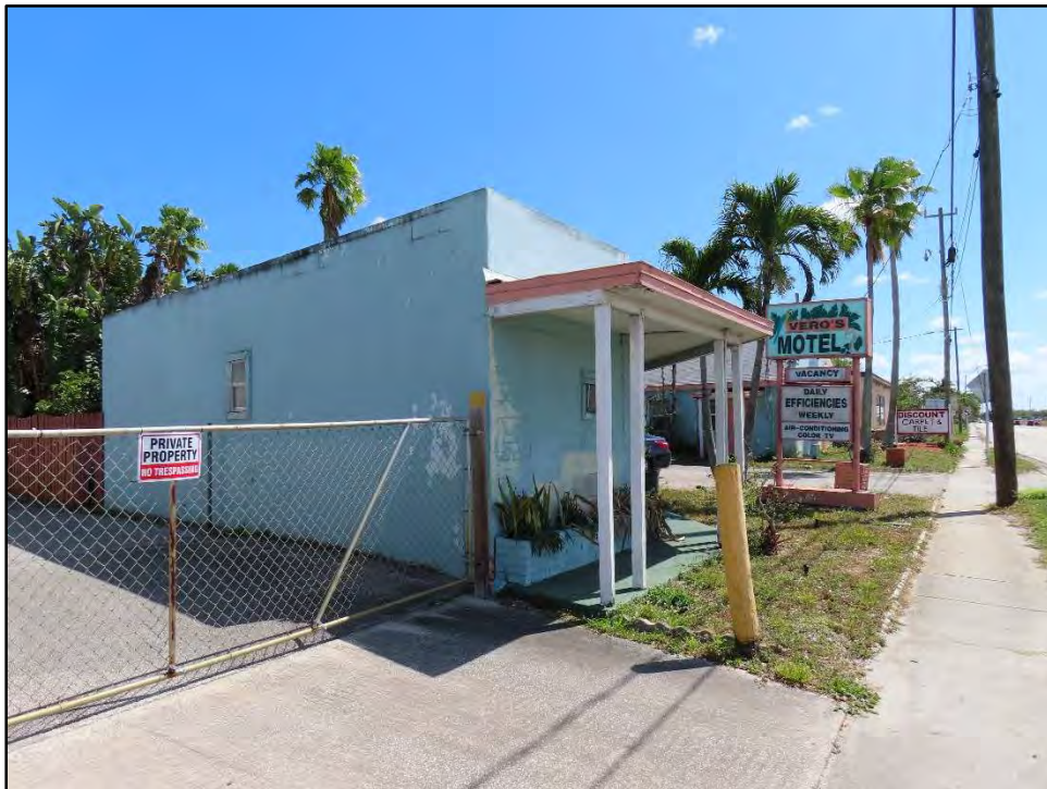
Figure 3: Vero's Motel Complex (8IR1904), c. 1951, facing South
