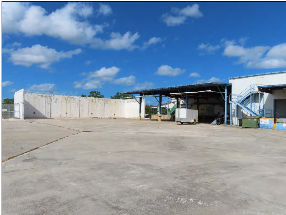
Figure 4: 2745 St. Lucie Avenue (8IR1894) Northwestern Additions, c. 1974, facing Northeast
