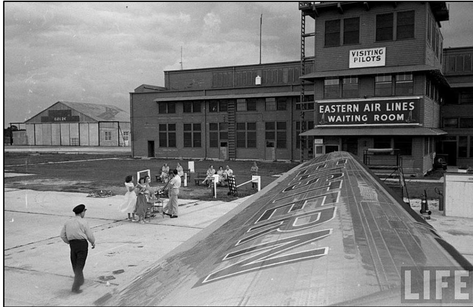
Figure 91: A 1949 Photo of the Terminal Building (Sunshine Skies)
