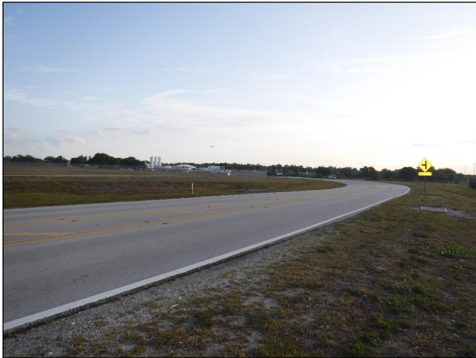
Figure 22: North Side of Aviation Blvd., where High Pressure Gas Line Runs Parallel to Road, facing East-Northeast
