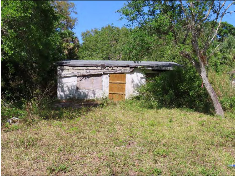
Figure 2: Representative Photo of Masonry Vernacular Camp Gordon Cottage; 1346 33 rd Street (8IR1884), c. 1950, Considered Ineligible, facing North
