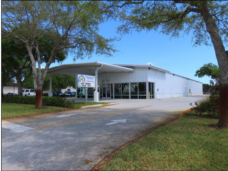
Figure 65: 2746 US Highway 1 (8IR1893), c. 1967, Considered National Register-Ineligible, facing Northeast
