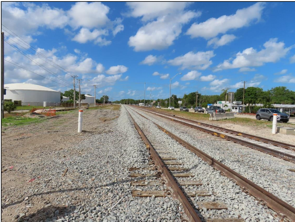
Figure 52: FEC Railway (8IR1497), c. 1892, Determined National Register-Eligible, From Intersection with Aviation Boulevard, facing North
