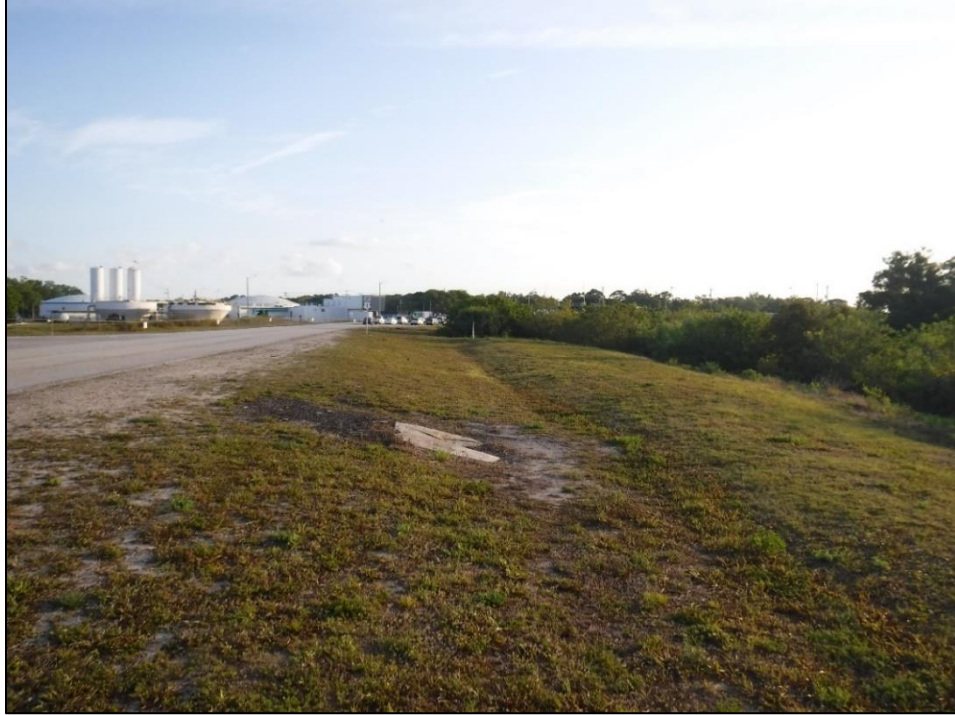
Figure 21: South Side of Aviation Blvd., with Storm Drain, Fiber Optic Cable, and Elevated Roadway Present, facing Northeast
