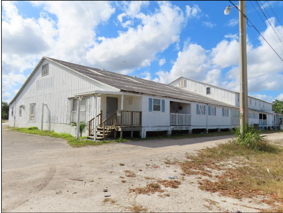
Figure 66: 2745 St. Lucie Avenue (8IR1894), c. 1950, Considered National Register-Eligible, facing Northwest
