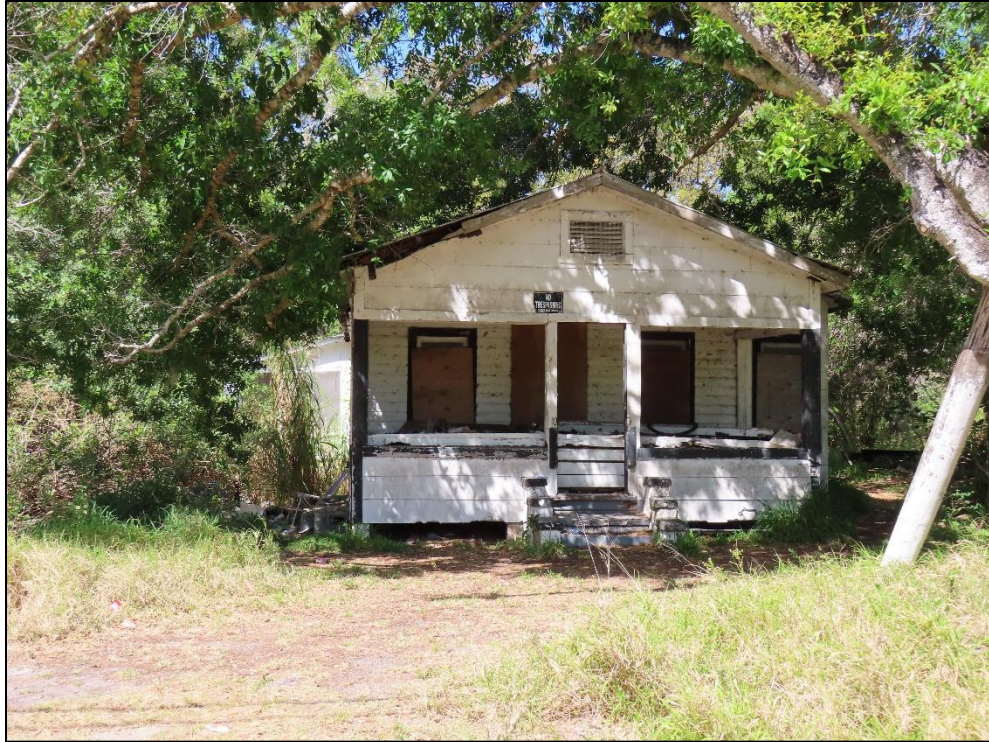
Figure 49: 1366 33 rd Street (8IR763), c. 1935, Considered National Register-Ineligible, facing North
