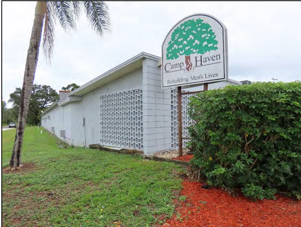
Figure 2: 3256 US 1 (8IR1883), facing Southeast
