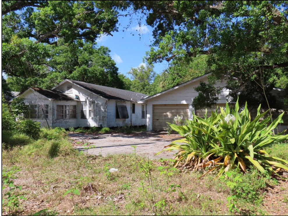
Figure 45: 1304-06 33 rd Street (8IR756), c. 1938, Considered National Register-Ineligible, facing Northwest
