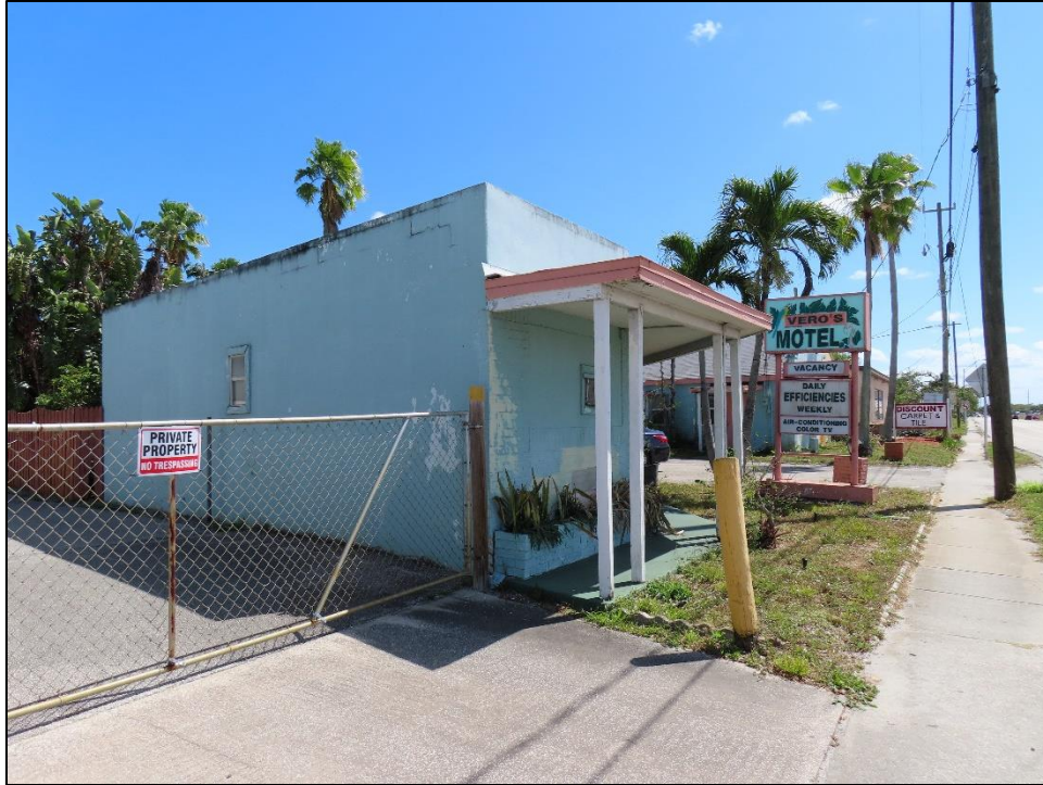
Figure 86: Vero's Motel Complex (8IR1904), c. 1951, Considered National Register-Ineligible, facing South
