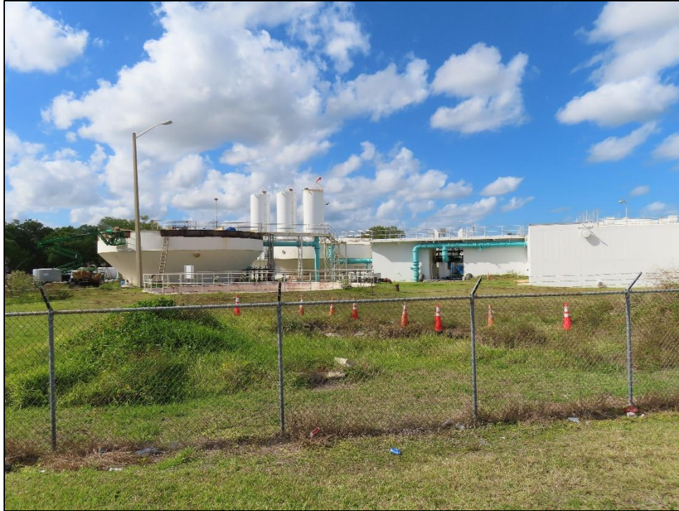
Figure 81: Vero Beach Water Treatment Facility (8IR1902), c. 1953, Considered National Register-Ineligible, facing North
