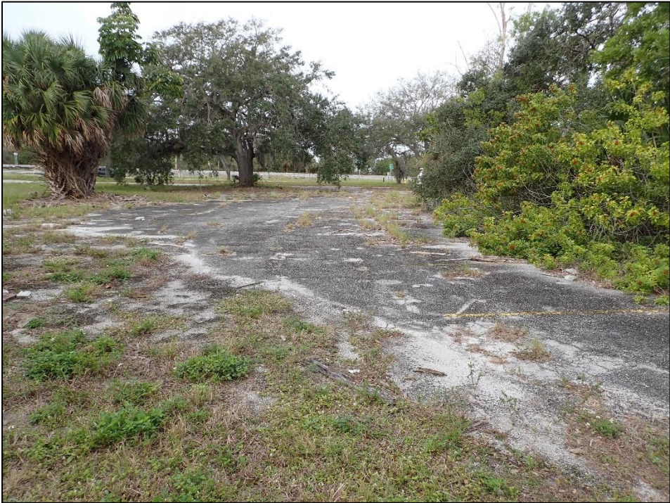
Figure 28: Northern Section of Proposed Pond 1A Showing Pavement, facing West
