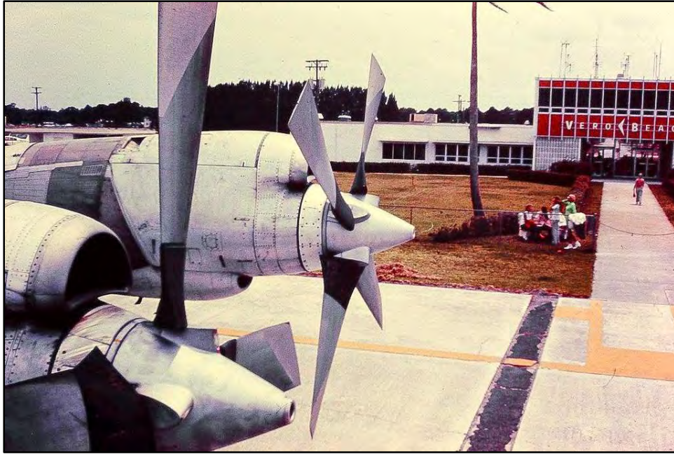
Figure 5: Undated Photo with the 1964 Terminal in the Background
