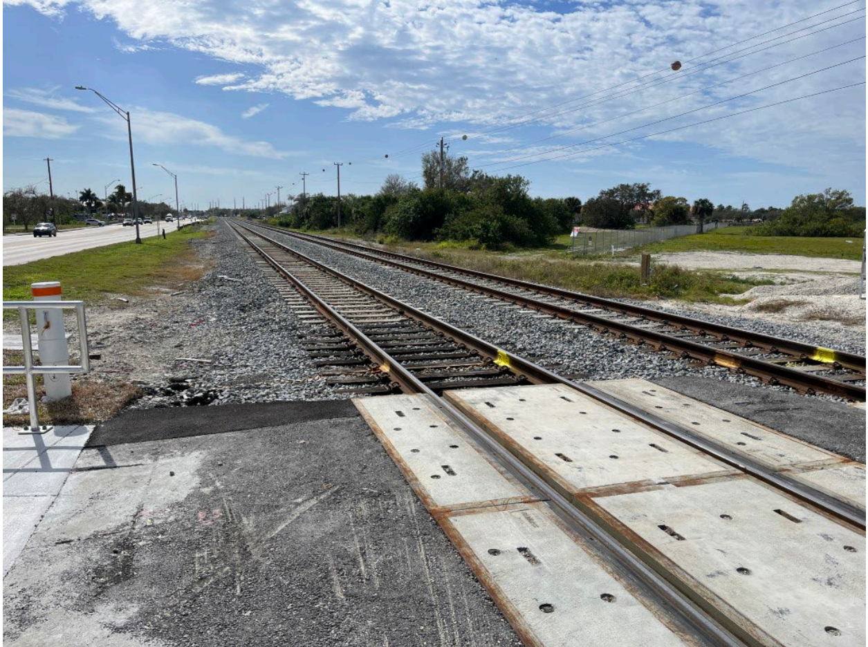
Photo 1. Map ID #1. FEC Railroad. Aviation Blvd crossing. Photo date 2/13/2024. View to south.
