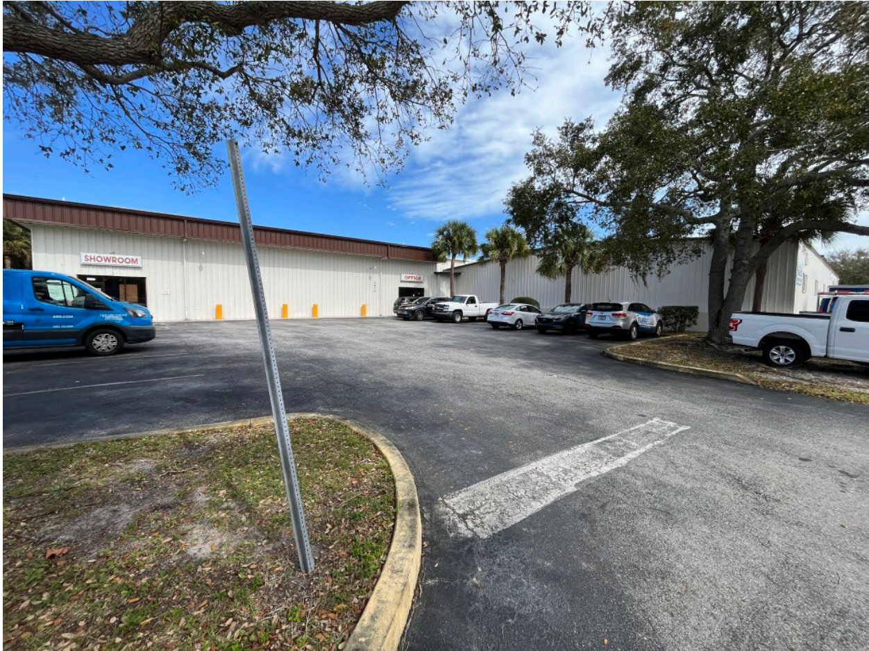
Photo 4. Map ID #4. Graves W C JR-Indian River Associates. Location of former USTs. Photo date 2/13/2024. View to north.
