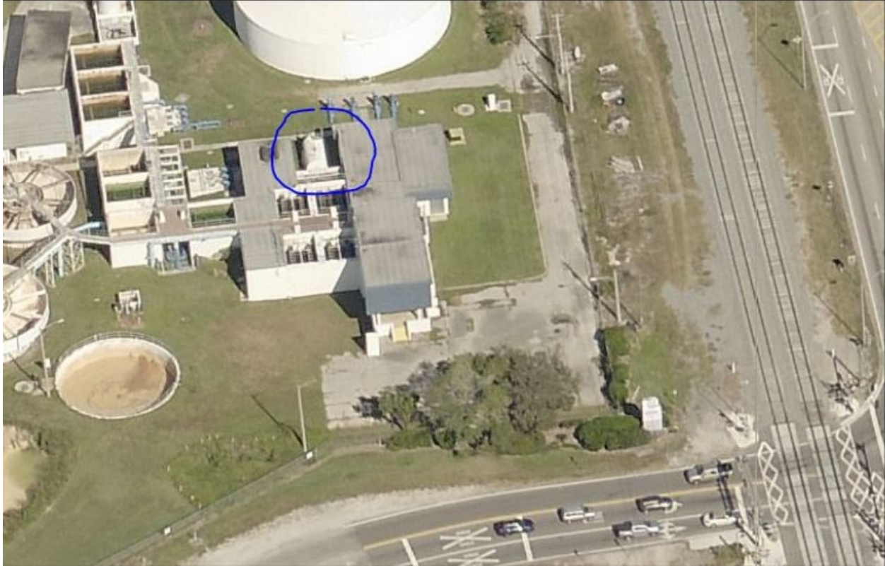
Vero Beach Water Treatment Plant (Map ID #5). 2023 oblique aerial photograph of the closest of the ASTs at the Vero Beach Water Treatment Plant to the project alternatives. Aviation Blvd in the foreground; FEC Railroad at right. View to north.
