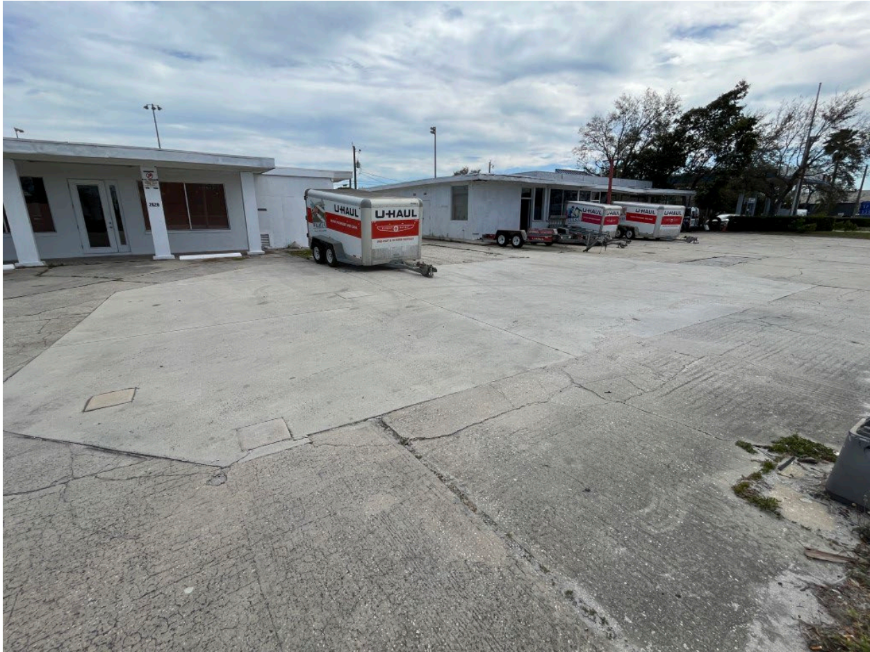
Photo 12. Map ID #12. Moran Service Station. Former gas station. Concrete patching for UST removal and abandoned monitoring wells are evident. Photo date 2/13/2024. View to southeast.
