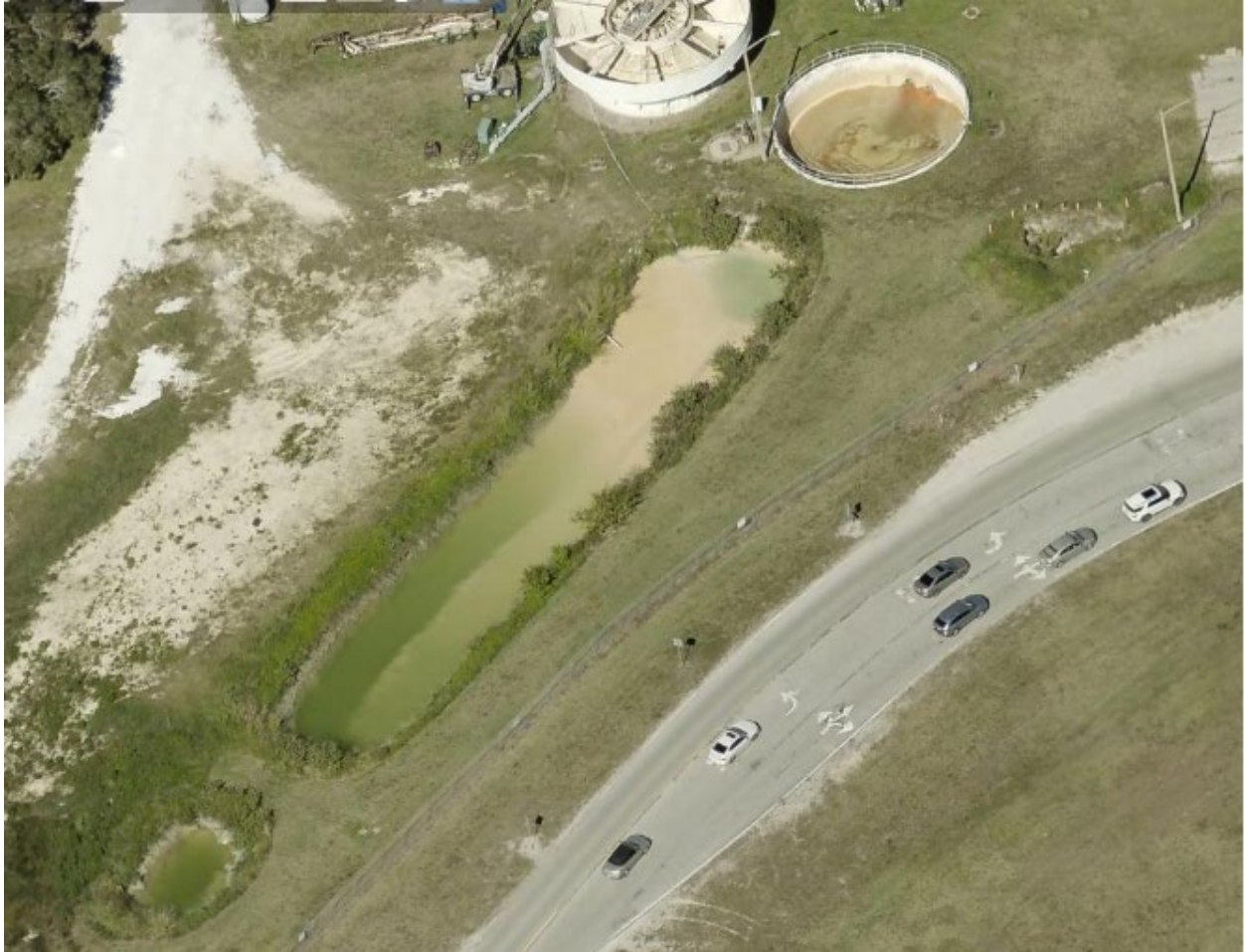
Vero Beach Water Treatment Plant (Map ID #2). 2023 oblique aerial photograph showing linear effluent pond that receives waste lime sludge. Oblique view to north. Aviation Blvd is in lower right
