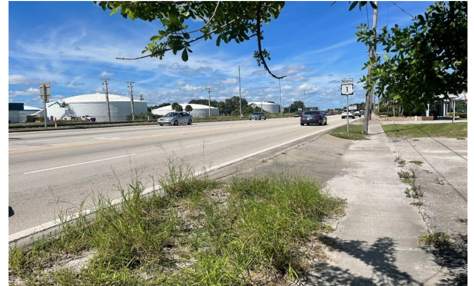
US-1 northbound at Aviation Blvd.
