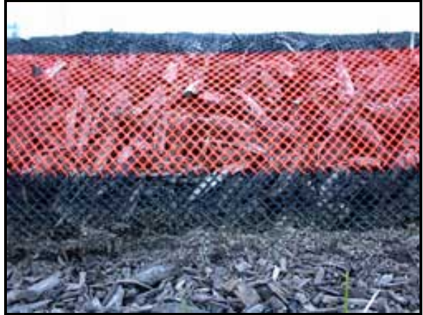
Detail of compost-filled mesh sock (Source: Filtrexx, 2006)
