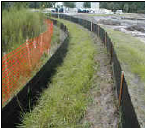
SRB prior to placement of mulch barrier
