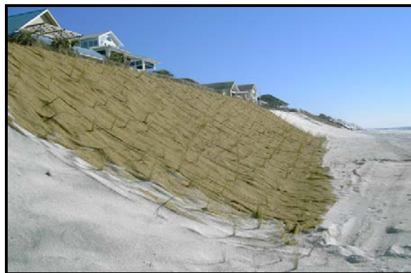
Armoring on beach with jute netting and salt-tolerant vegetation (Source: Foundation Technologies, 2006)
