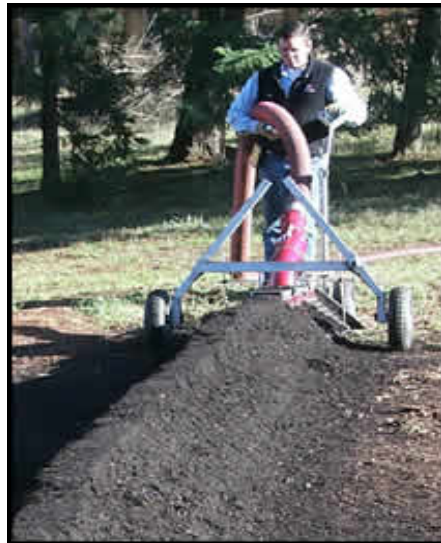
Installation of compost berm (Source: Rexius, 2006)
