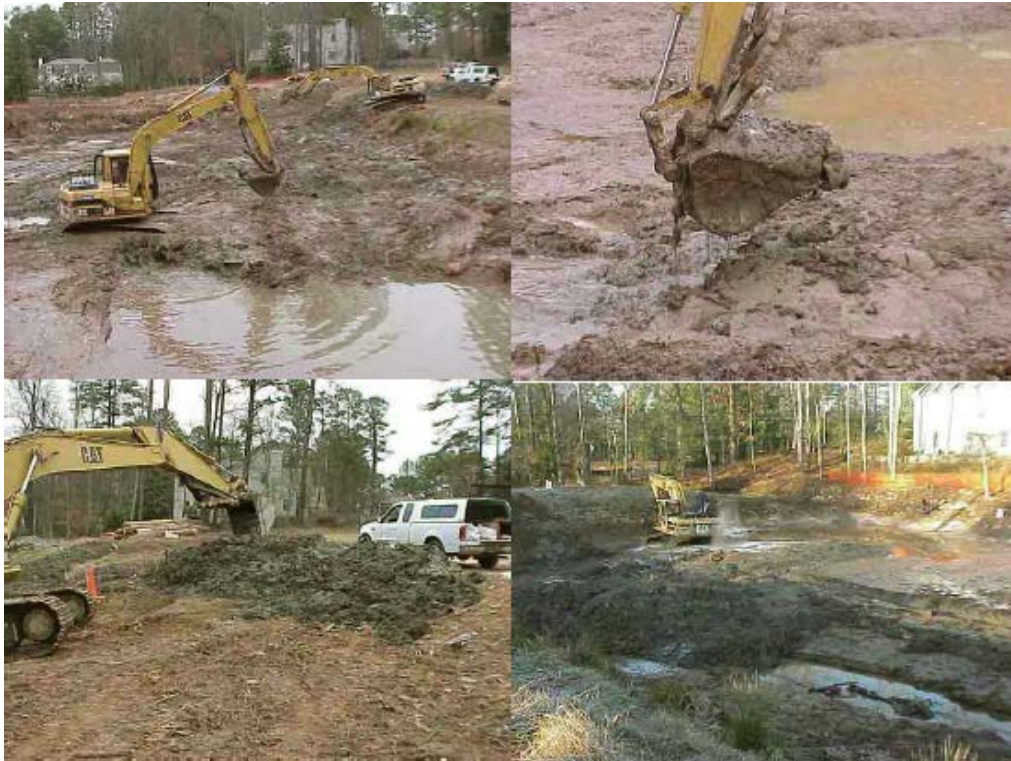
Figure AIII-28: Polymer-enhanced Mud and Sediment Removal.
