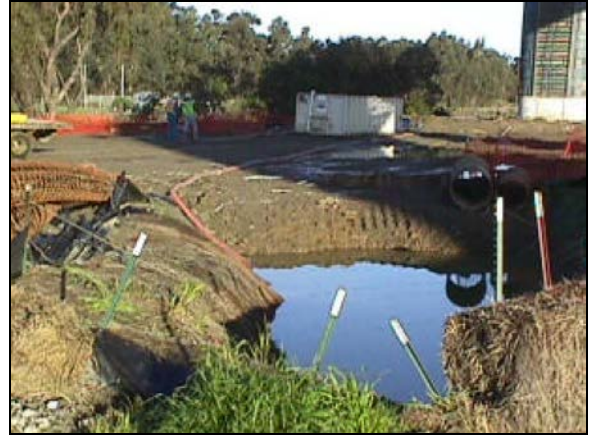
Sediment Trap (Source: http://www.mnerosion.org )
