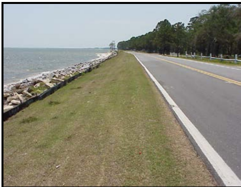
Armoring in place, one year later
