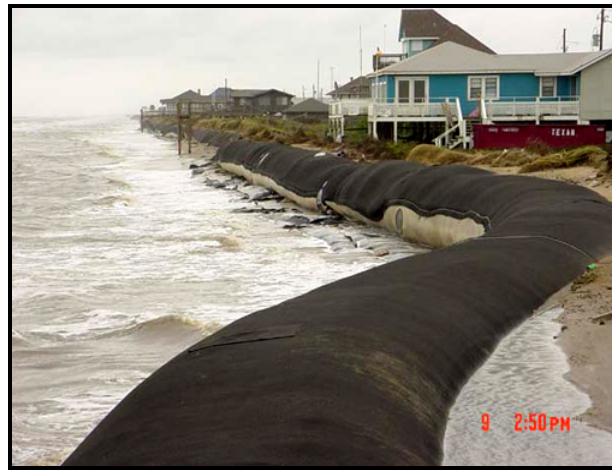
Sandsack, sand-filled tubular geotextile (Source: Surfrider Foundation, 2006)
