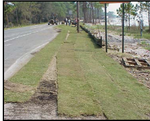
Final placement of sod
