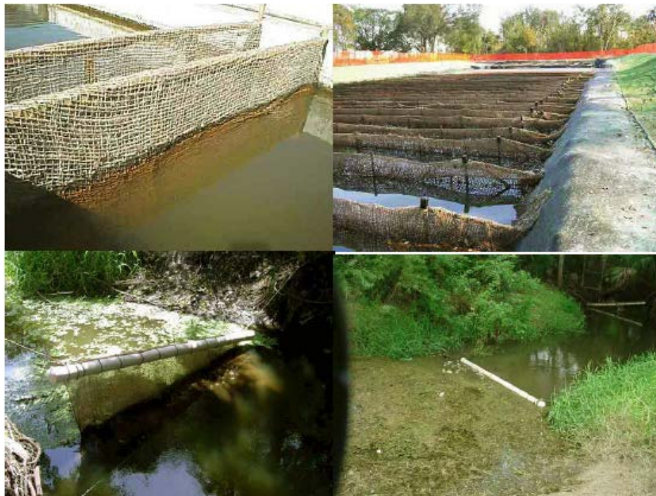
Figure AIII-25: Polymer-enhanced Particle Curtains.
