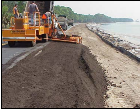
Placement of compost mulch layer
