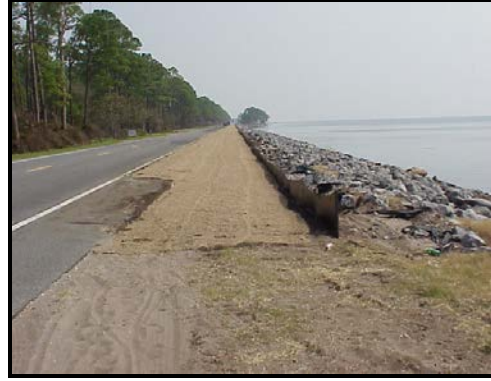
Placement of jute fiber erosion control blanket
