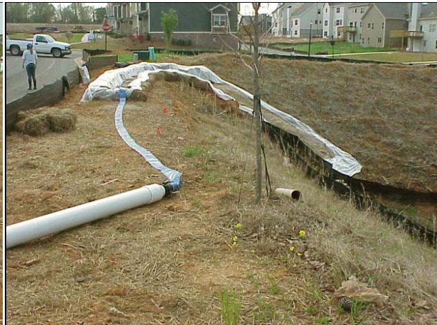
Figure AIII-3: The water was pumped through the pipe mixers and down a jute lined ditch.
