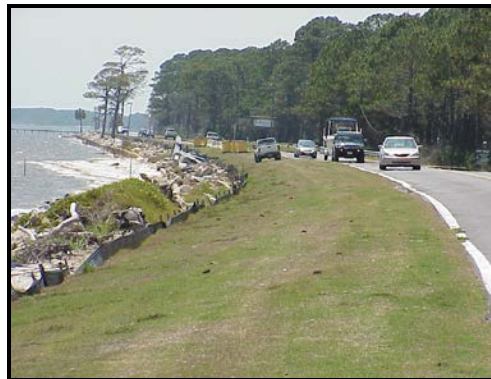
Roadway and shoulder successfully protected
