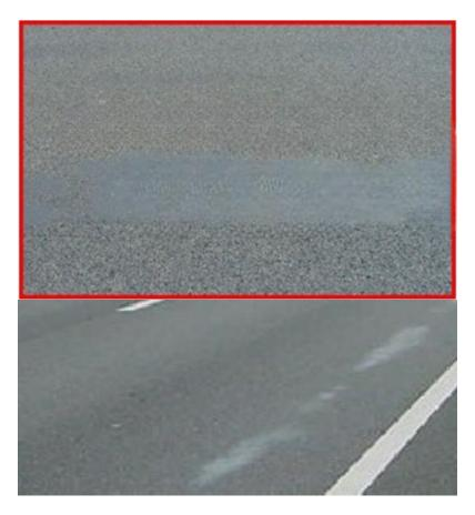
**SLIPPAGE**- The movement between layers when none should exist. Picture illustrates classical U pattern.
