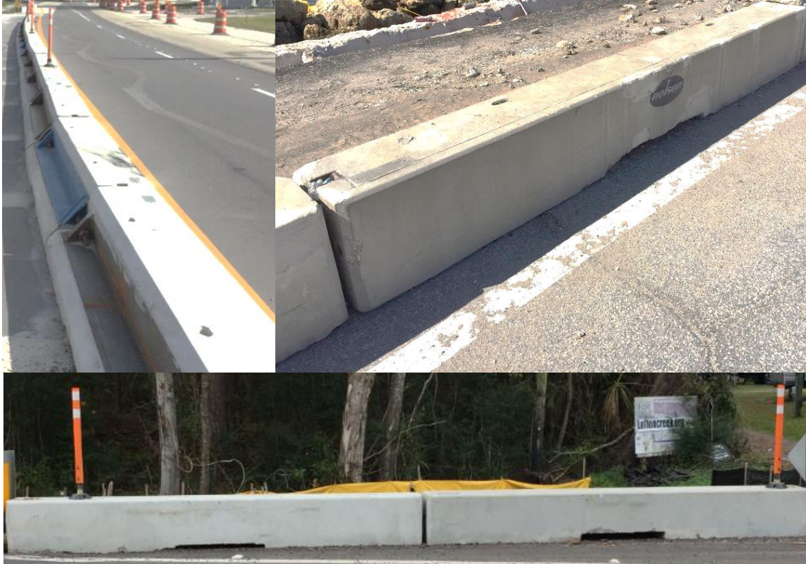
Figure 1: Examples of Acceptable Low-Profile Concrete Barrier
