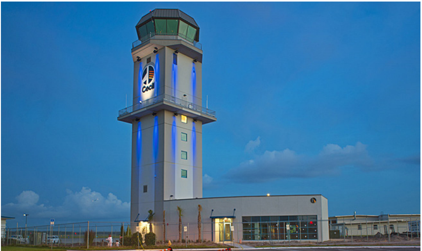
New Cecil Control Tower, Cecil Spaceport Source: Cecil Spaceport
