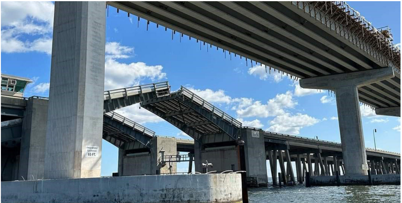
Indian River Bridge Reconstruction (03/30/23). Source: Space Florida
