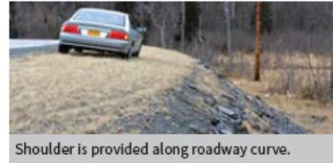
Shoulder is provided along roadway curve.
