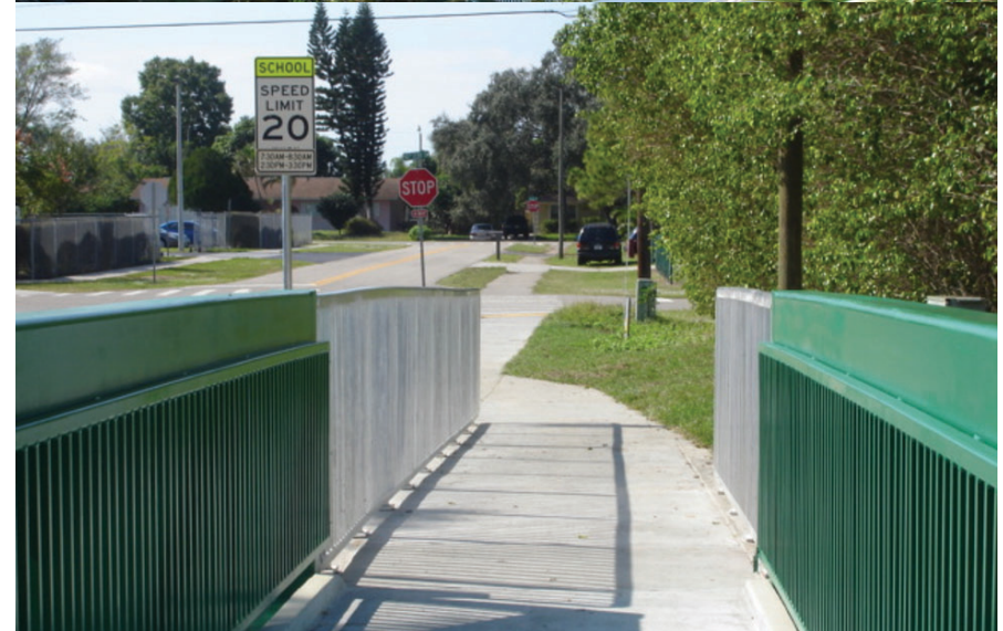
SRTS-Funded Pedestrian Bridge in Collier County
