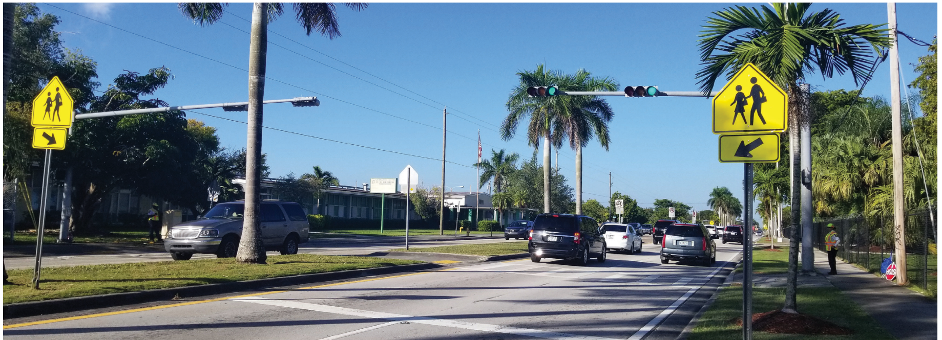
Upgraded Signs, Pedestrian Push Buttons and Crosswalk at a School Crossing
