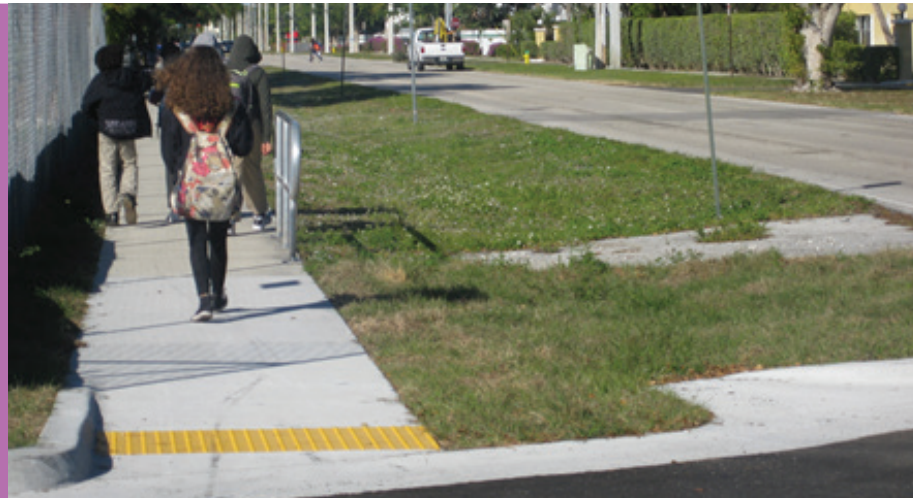
Figure 18: New Sidewalk near Deerfield Beach Elementary School, Broward County, FDOT District 4
