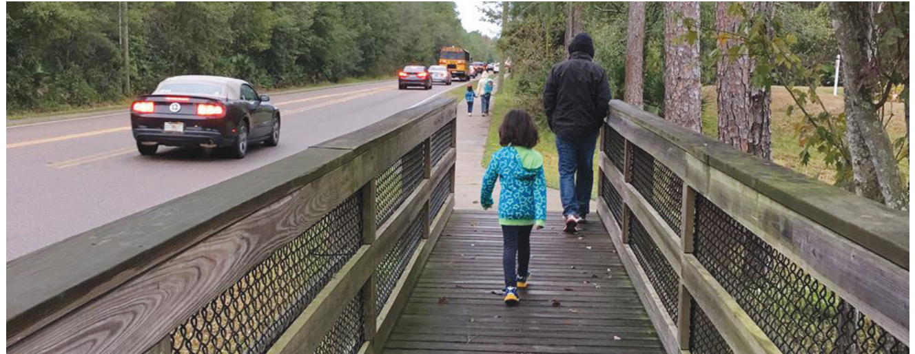
Figure 14: New Sidewalk Serving Bryant Elementary School and Farnell Middle School, Hillsborough County, FDOT District 7
