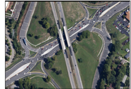
Figure 1. Harrodsburg Road at KY 4 DCD Interchange, Lexington, KY
