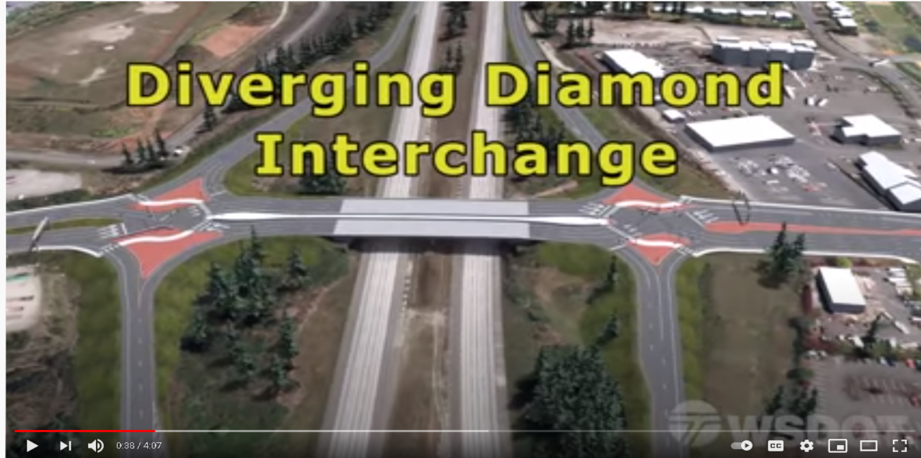
Diverging Diamond Interchange comes to Washington State
