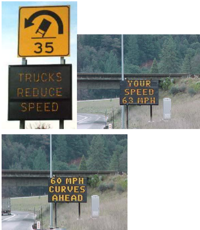
FIGURE 49 Dynamic curve warning system.
