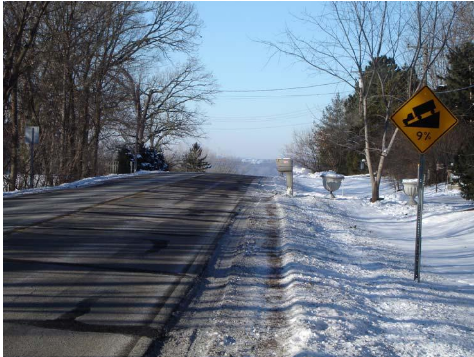
FIGURE 53 Advance warning of a steep grade.
