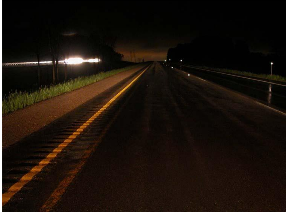
FIGURE 34 Painted edgeline rumble strips.
