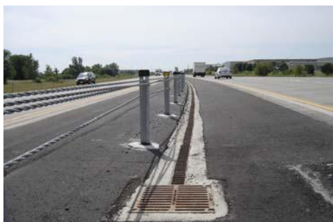
FIGURE 56 Continuous drainage system.
