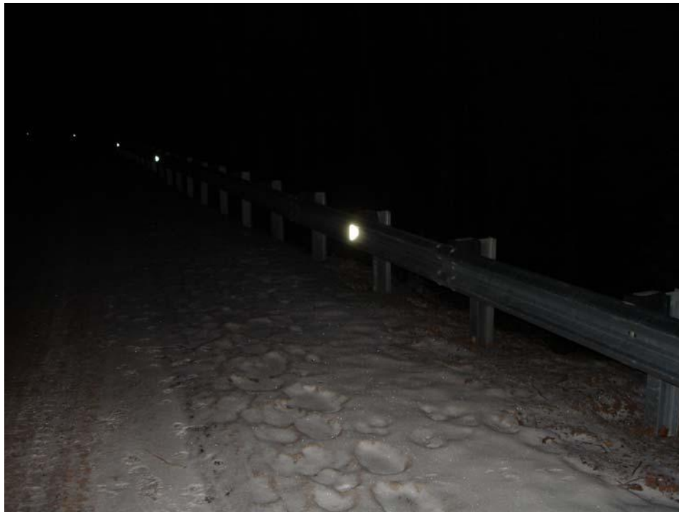
FIGURE 52 Delineation with reflectors on barrier.
