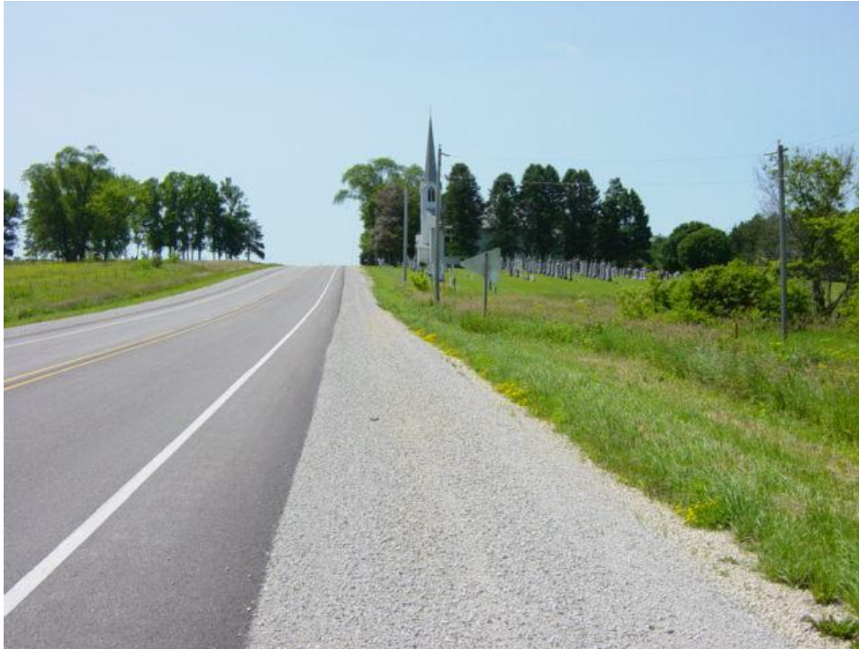
FIGURE 9 Pavement edge drop-off.
