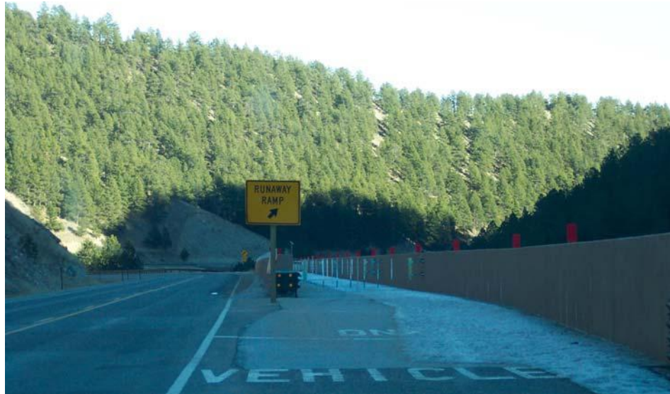
FIGURE 55 Truck escape ramp.
