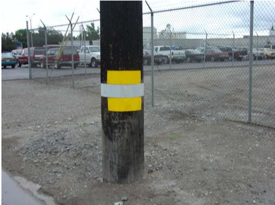
FIGURE 69 Reflective sheeting on utility poles.
