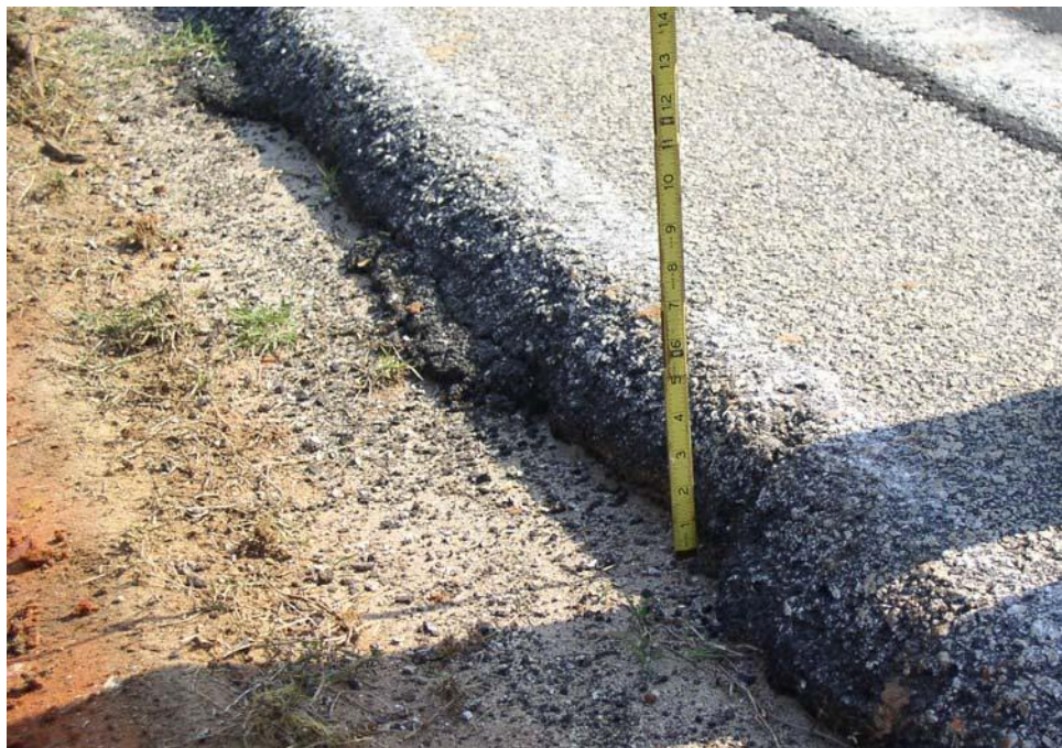
FIGURE 9 Pavement edge drop-off.
