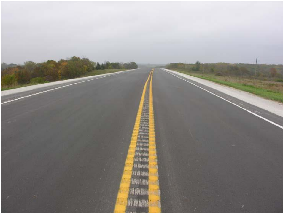
FIGURE 33 Centerline rumble strips.
