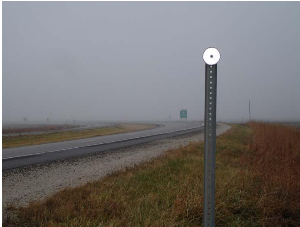
FIGURE 30 Post-mounted delineators.
