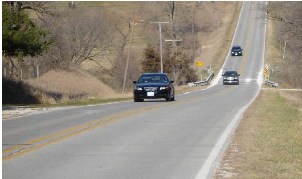
FIGURE 13 Vehicle shying towards the centerline on a narrow bridge.
