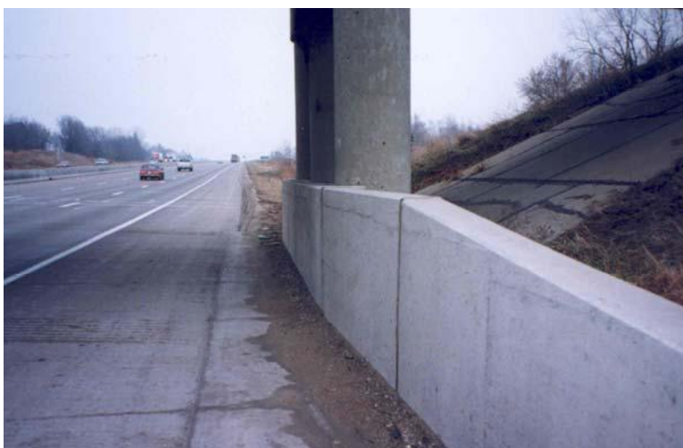
FIGURE 39 Shielding fixed objects with barrier.
