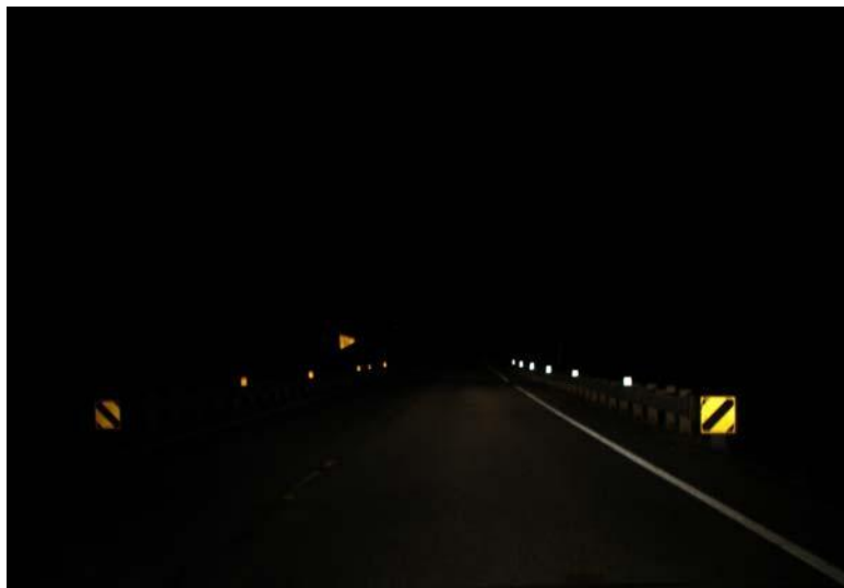
FIGURE 42 Reflector tabs on guardrail.
