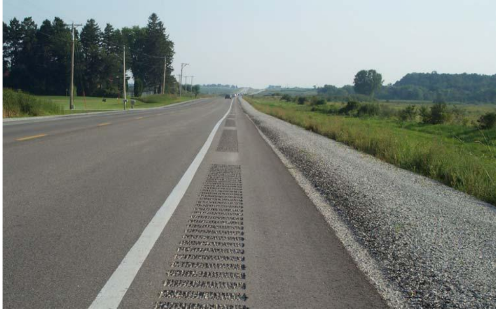
FIGURE 33 Centerline rumble strips.
