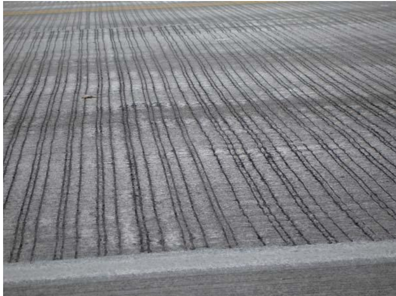
FIGURE 63 Transverse grooving to improve surface drainage and friction.
