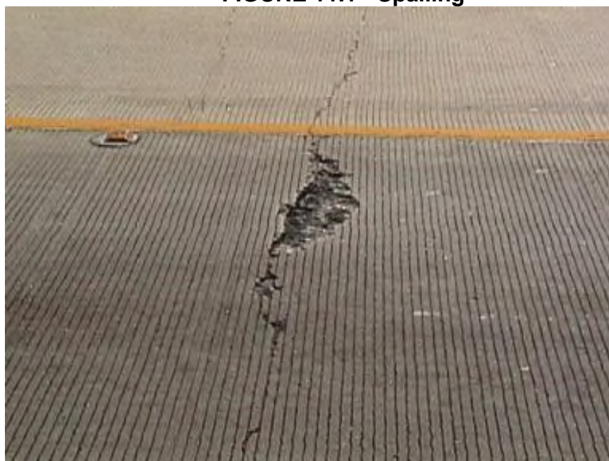
FIGURE 11.1 - Spalling
