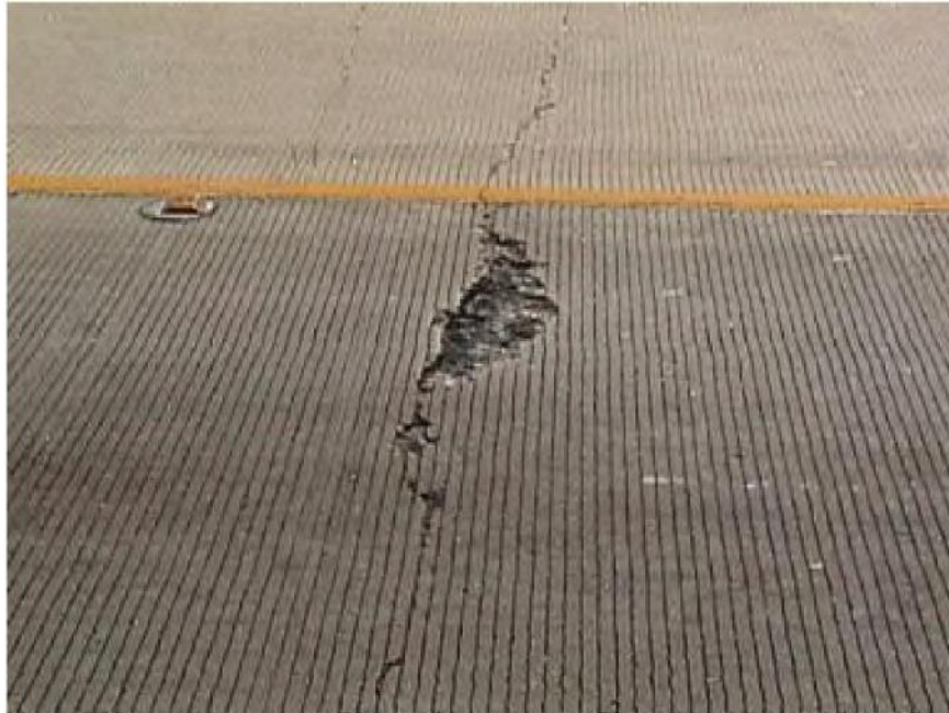
FIGURE 11.1 – Spalling
