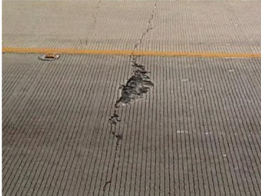
FIGURE 11.1 – Spalling
