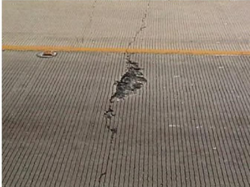
FIGURE 11.1 – Spalling
