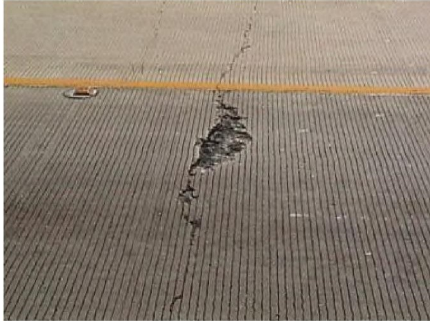
FIGURE 11.1 – Spalling
