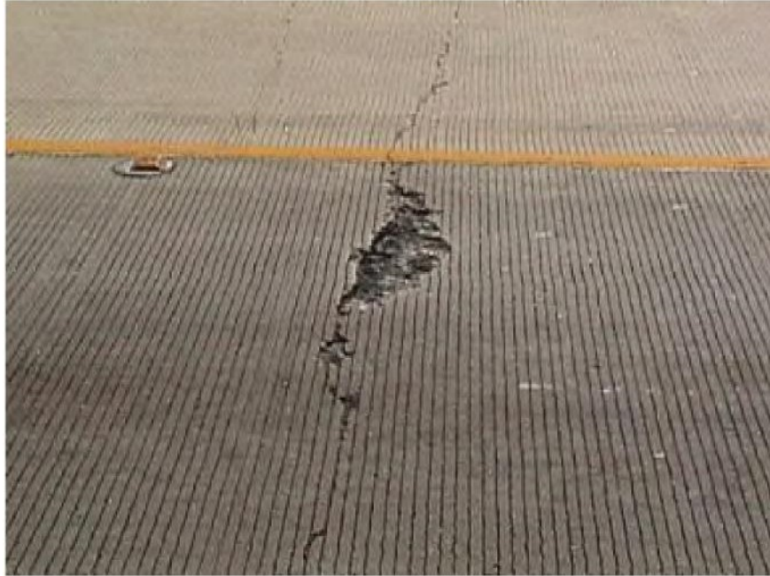
FIGURE 11.1 – Spalling
