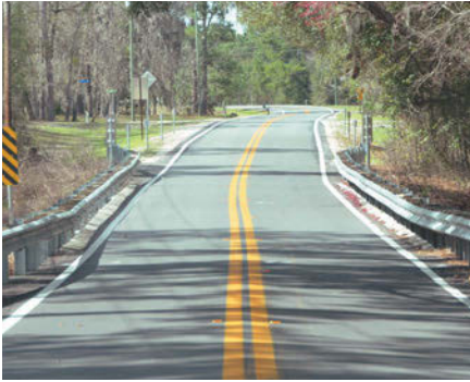
District 2 Honorable Mention: V.E. Whitehurst & Sons for their project on 180th Street from US 129 to CR 49 in Suwannee County. Tonnage: 7133.80, Lane Miles: 9.05
