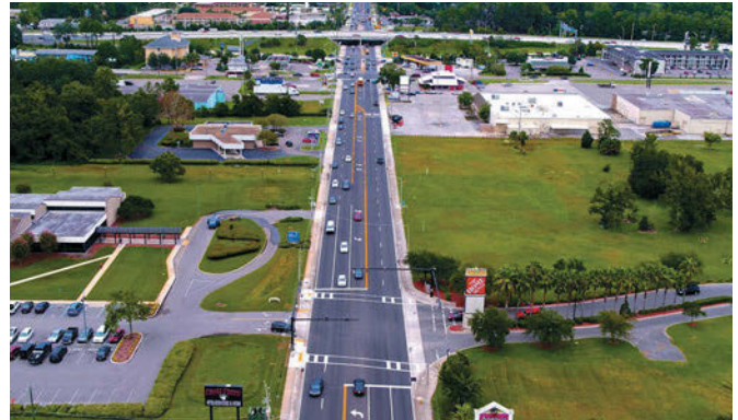
District 2: Duval Asphalt Products, Inc. for their project on SR 103 (Lane Ave.) from Normandy Blvd. to the railroad tracks at US 90 in Duval County. Tonnage: 7897, Lane Miles: 6.0
