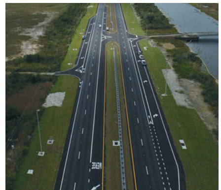
District 6: General Asphalt Company, Inc. for their project on SR 997/Krome Ave./NW 177th Ave. north of 8th Street from MP 0.657 to MP 5.121 in Miami-Dade County. Tonnage: 29441, Lane Miles: 17.9
