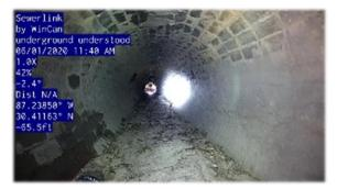
Dry pipes can be both evaluated and documented with stationary cameras. The illumination and zoom features of these cameras allows for more detailed inspections than can be accomplished by simply looking into the pipe. The software supplied with the camera allows the reviewer to enter documentation while performing the inspection. The limitation
