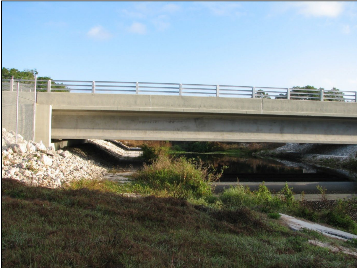
Figure 17 – 1 Bridge with Shelves for Wildlife
