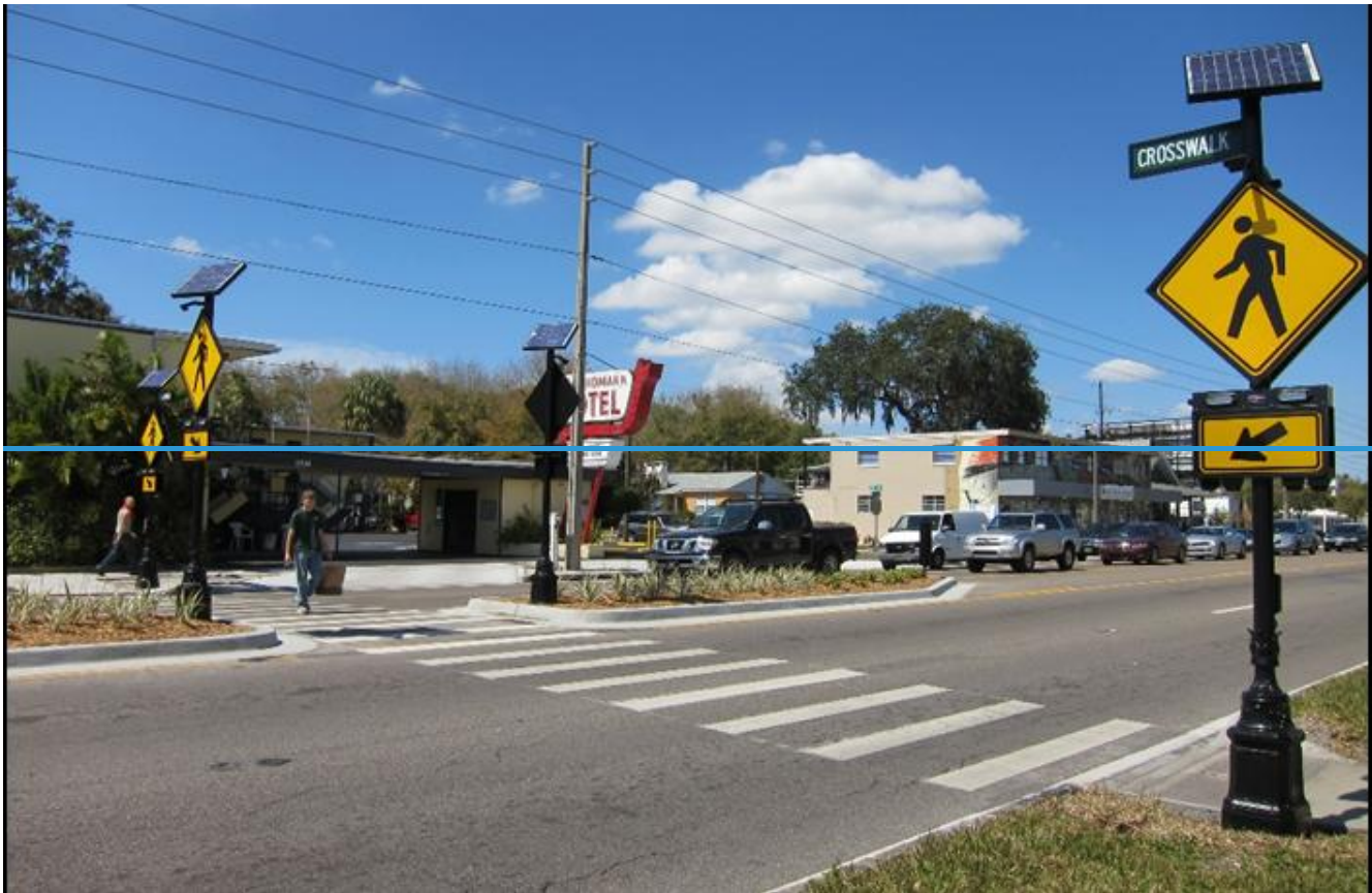
Figure 8-8 Pedestrian Median Refuge with Rectangular Rapid Flashing Beacons (RRFB)
