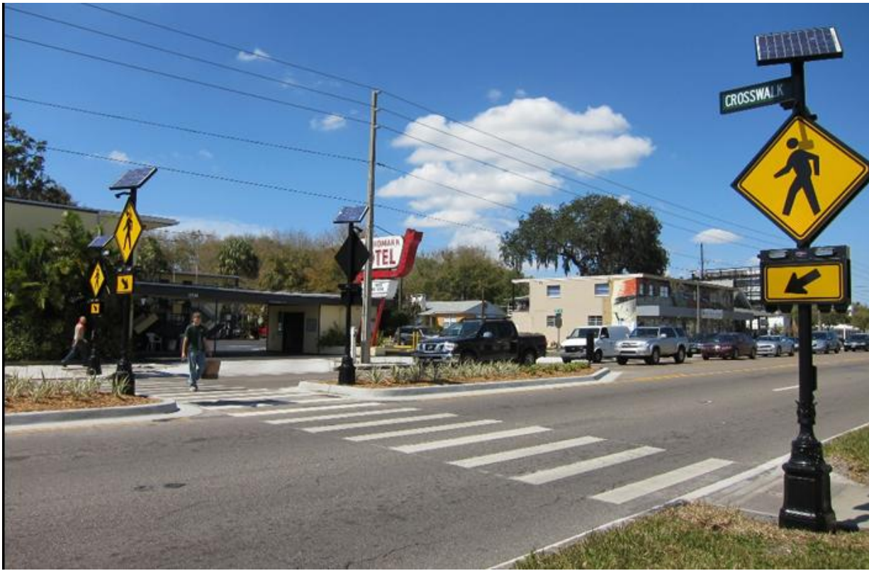
Figure 8-8 Pedestrian Median Refuge with Rectangular Rapid Flashing Beacons (RRFBs)
