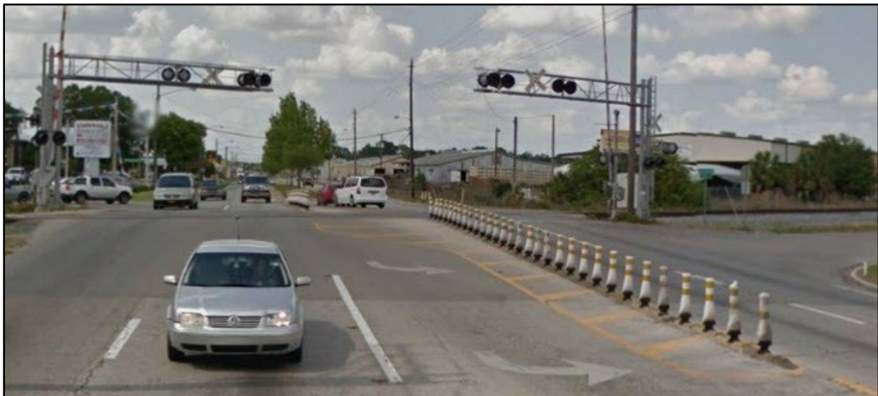
Alexander Street, SR 39A, Plant City, FL 1
