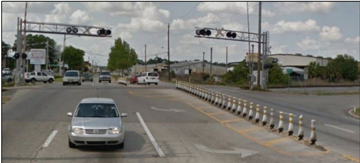
Alexander Street, SR 39A, Plant City, FL 1
